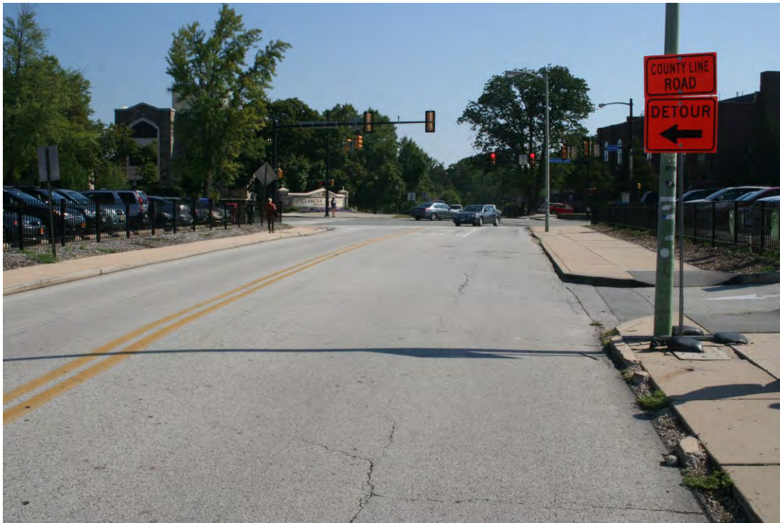
Description: Northbound on Ithan Avenue (approaching intersection)
