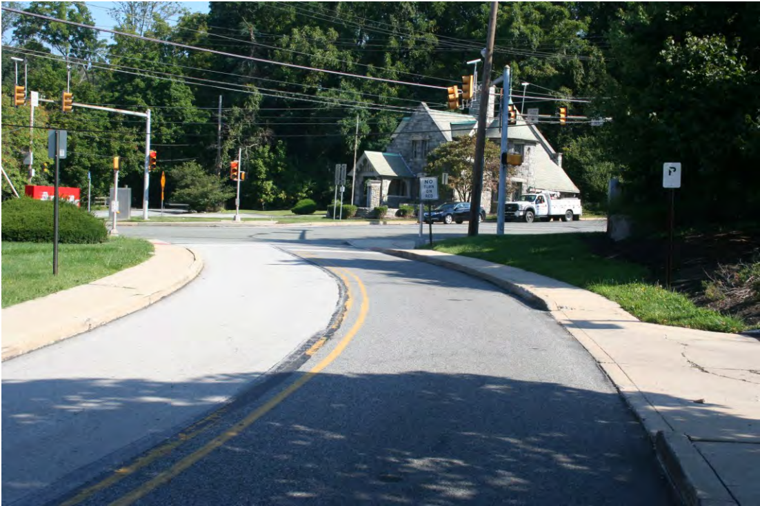
Description: Northbound on Aldwyn Lane (approaching intersection)
