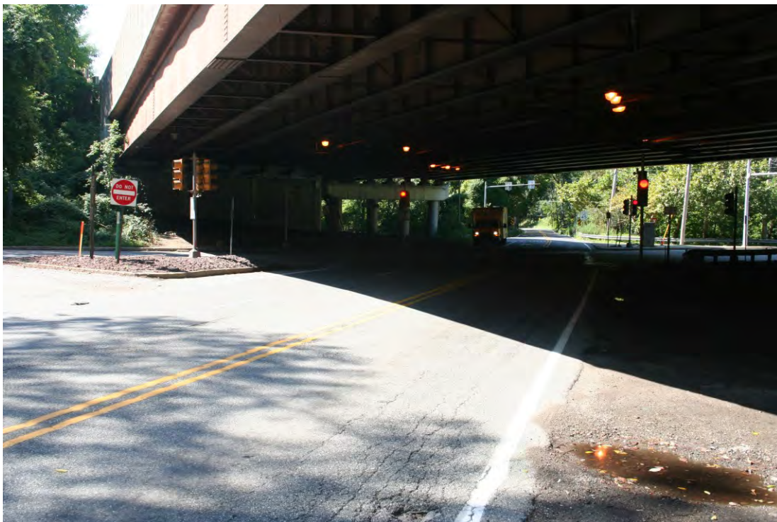
Description: Southbound on Sproul Road (approaching intersection)
