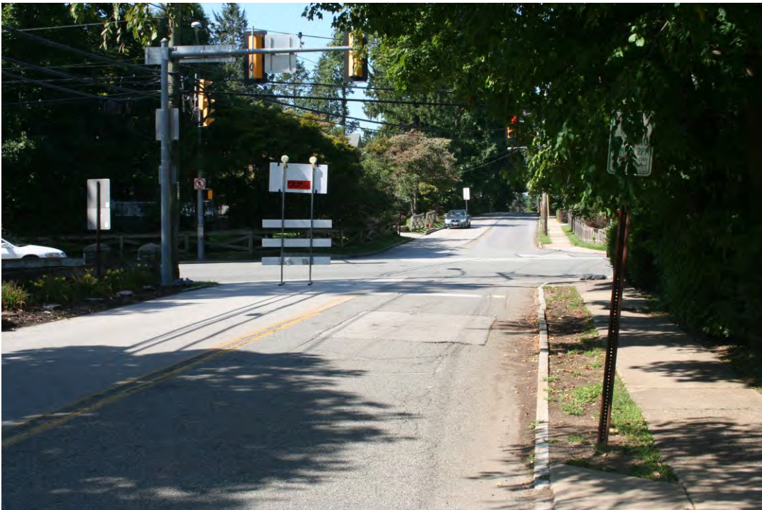
Description: Southbound on Lowrys Lane (approaching intersection)
