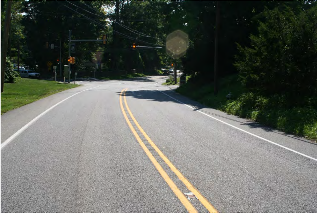
Description: Description: Eastbound on Conestoga Road (approaching intersection)
