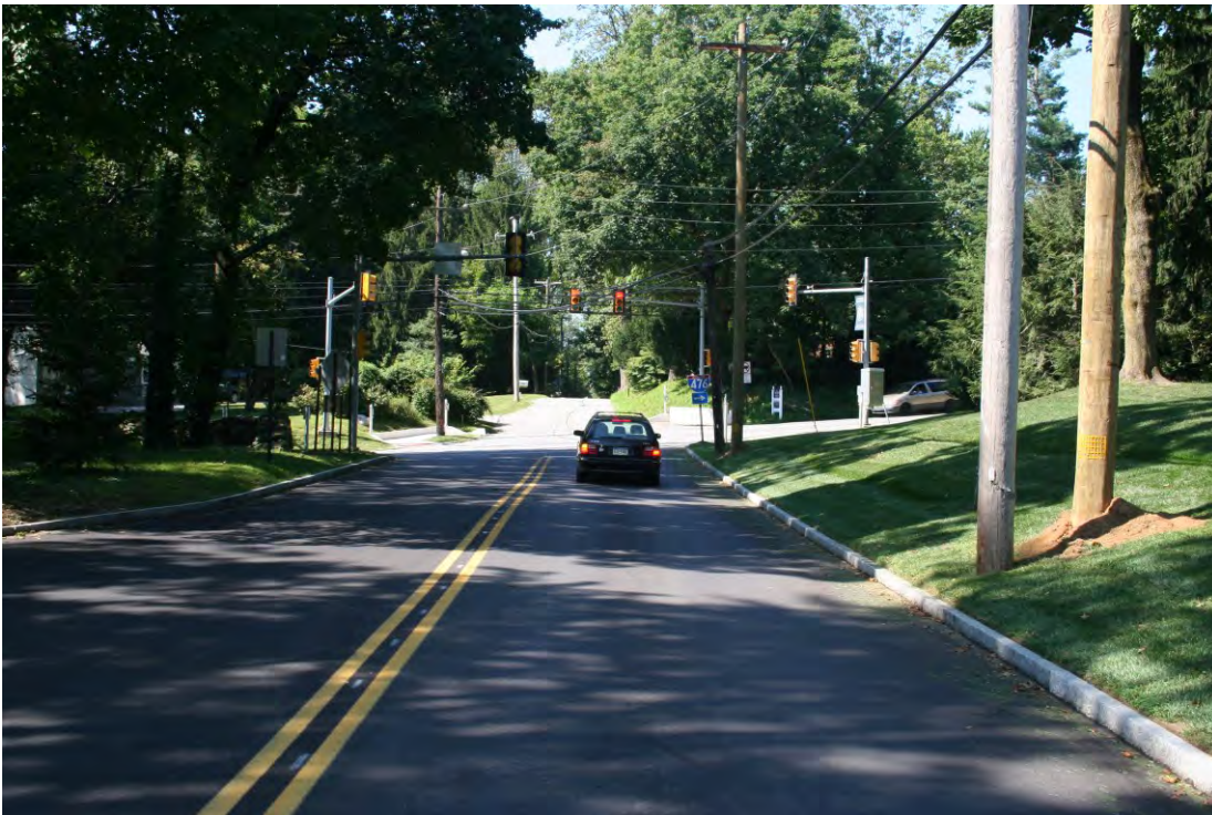
Description: Southbound on Ithan Avenue (approaching intersection)
