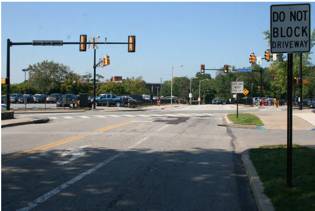
Description: Southbound on Ithan Avenue (approaching intersection)
