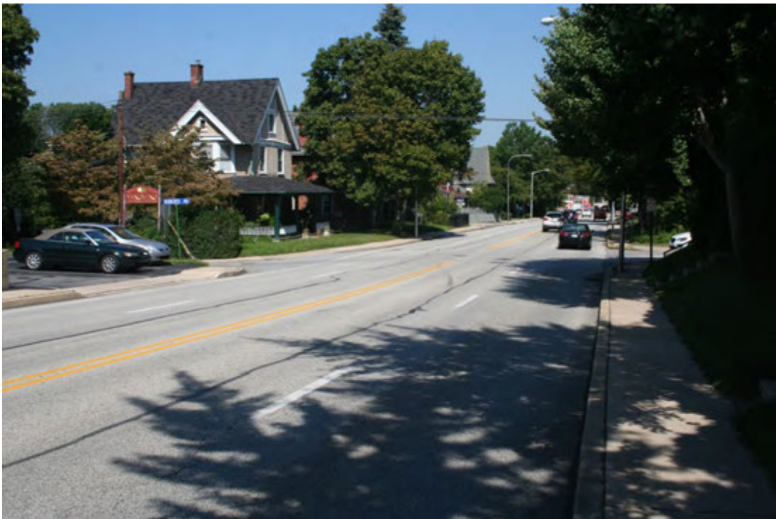
Description: Westbound on County Line Road (approaching intersection)
