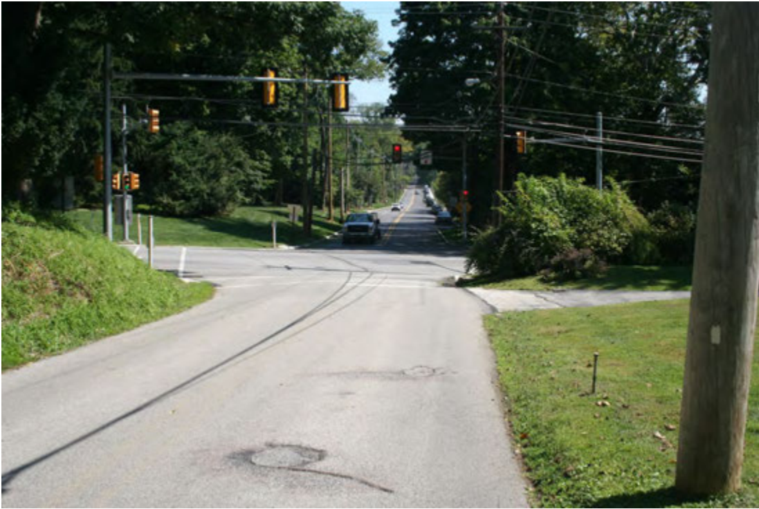
Description: Northbound on Ithan Avenue (approaching intersection)
