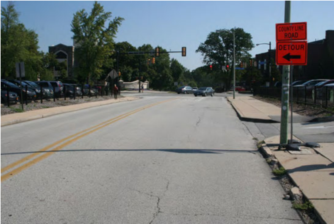
Description: Northbound on Ithan Avenue (approaching intersection)
