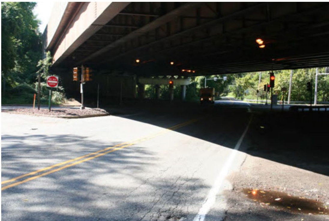
Description: Southbound on Sproul Road (approaching intersection)
