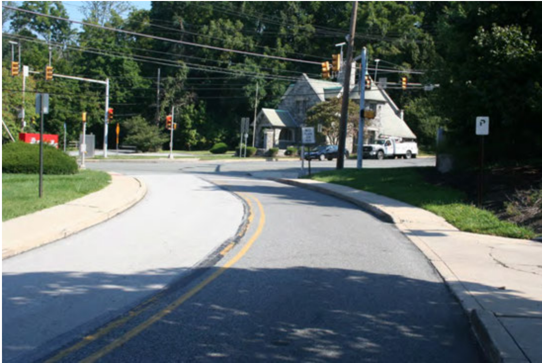
Description: Northbound on Aldwyn Lane (approaching intersection)
