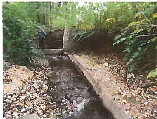
Figure 1: Photo of exposed sanitary sewer line
