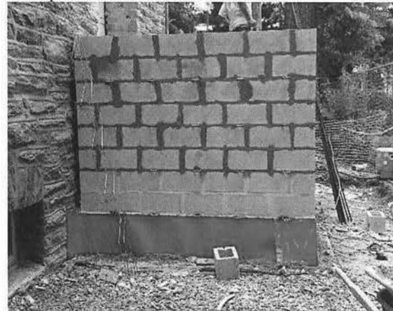
CMU installation for elevator shaft
