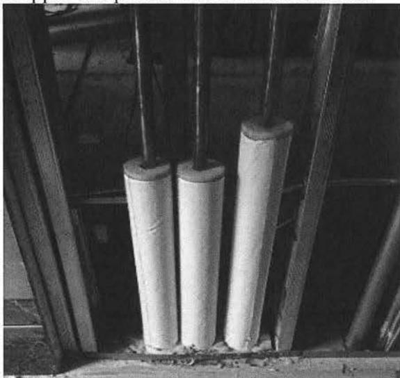
Insulated pipes and sealed floor penetrations
