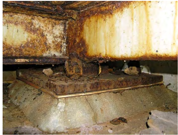
Right Bearing – North Abutment -Expansion
