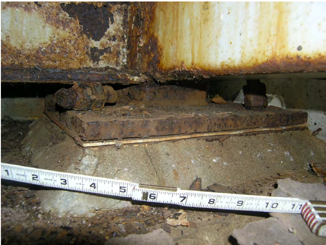
7) Right expansion bearing at far (north) abutment—broken inside anchor bolt
