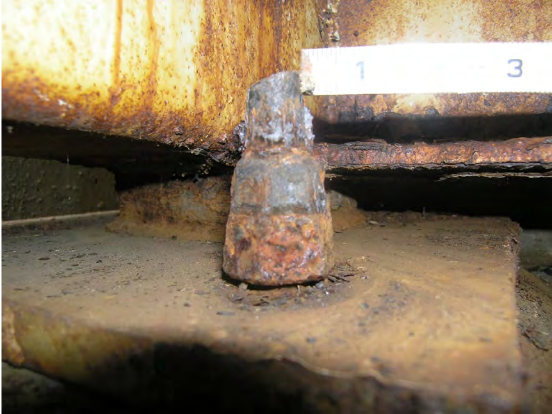
8) Left expansion bearing at far (north) abutment –section loss to inside anchor bolt nuts
