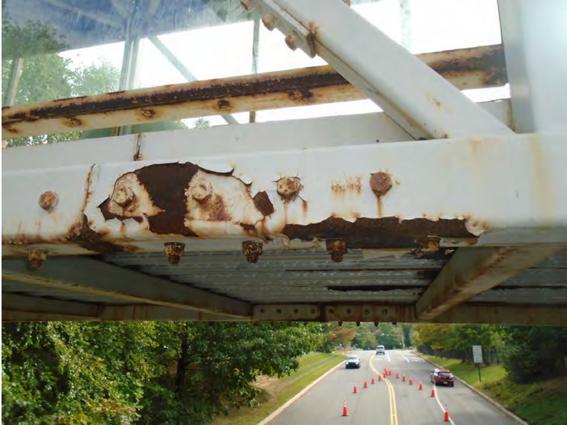
1) Typical rust and peeling paint at midspan splices—bottom chord shown
