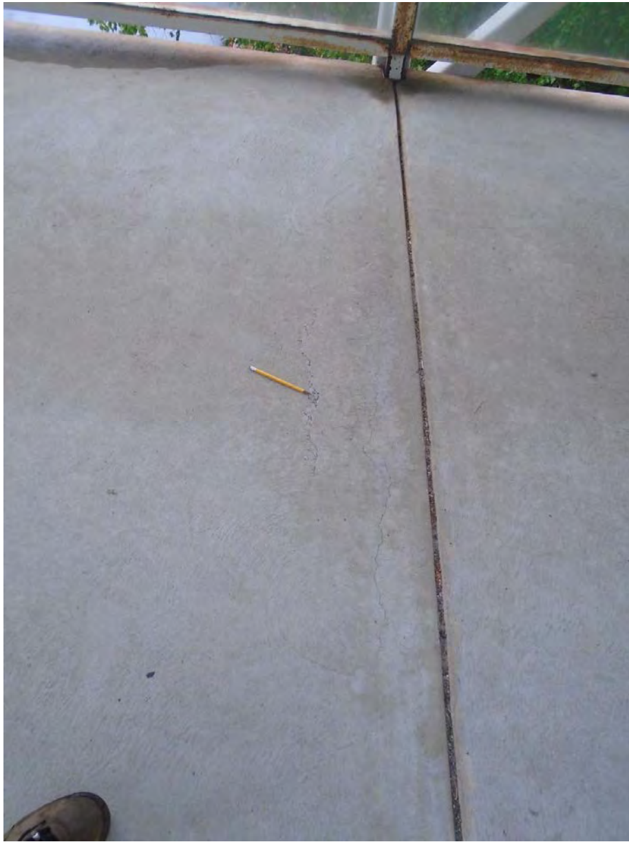
26) Fine transverse crack and small delamination in walking surface at Panel Point 8
