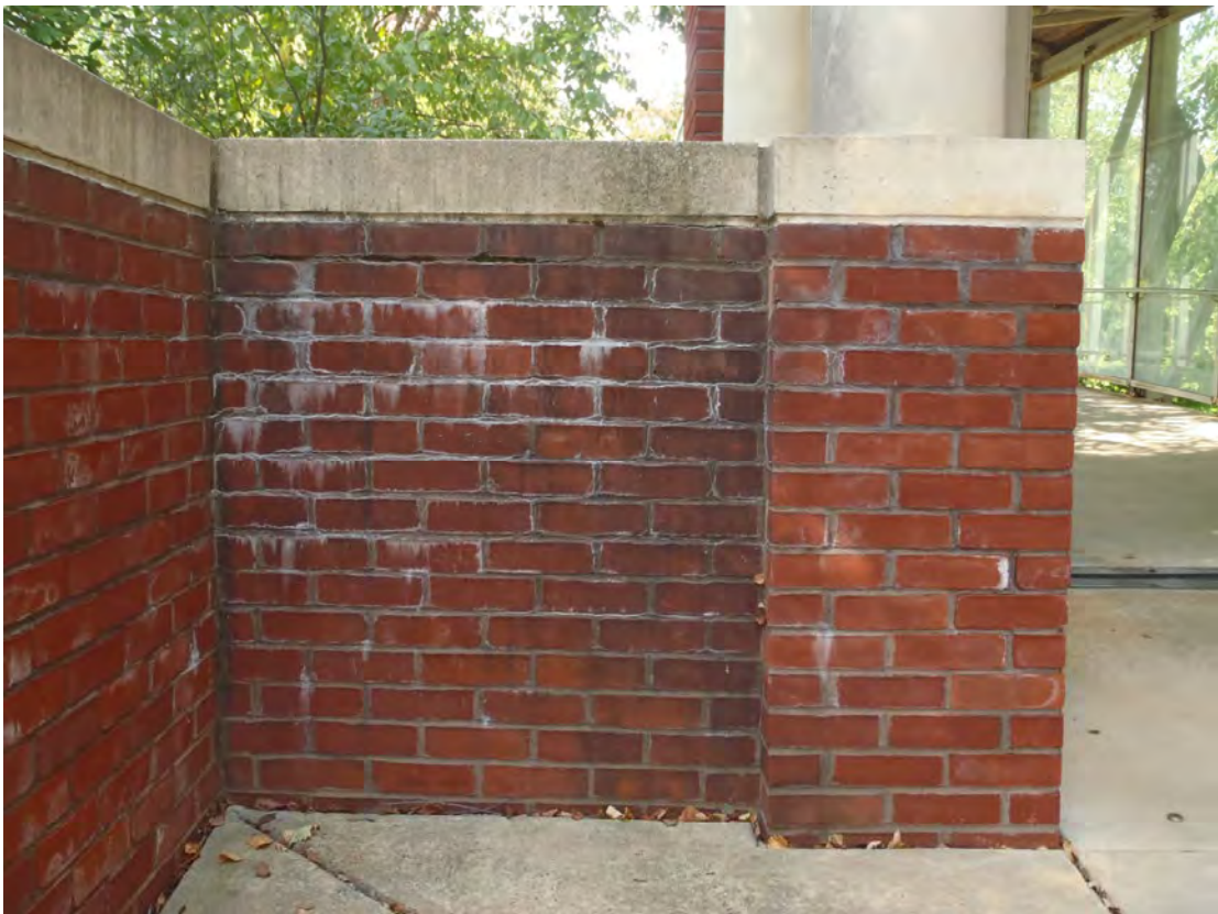
21) Wing Wall B, rear face parapet—Typical condition, areas of missing pointing and efflorescence
