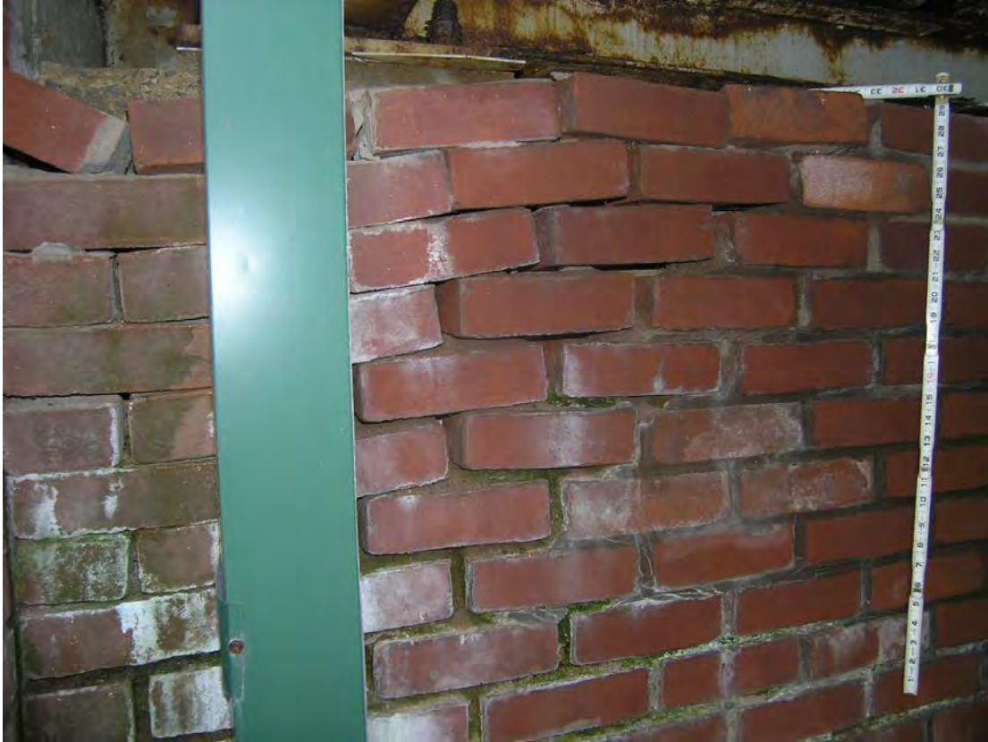
13) Left side of far (north) abutment—loose and unstable brick with missing pointing
