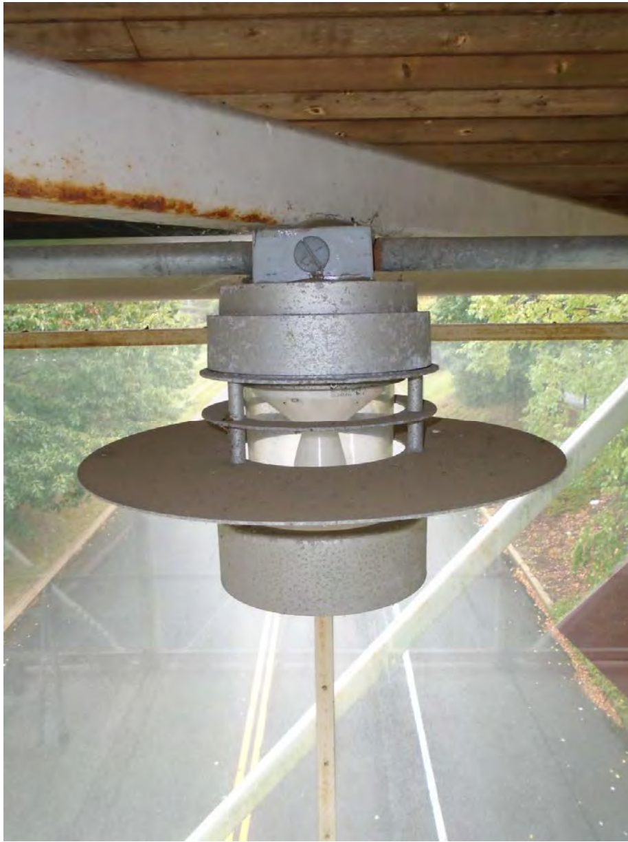
30) Typical light fixture attached to top diagonal brace
