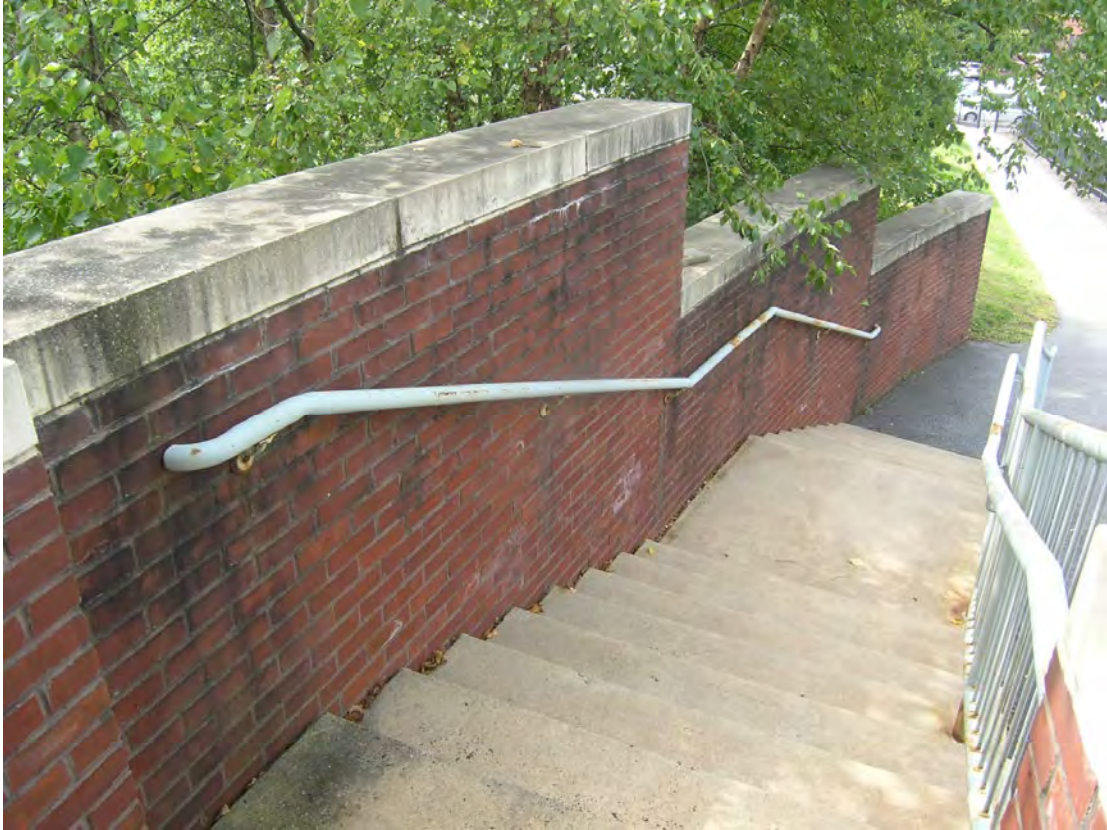
22) Wing Wall C rear face parapet, handrail and stairs.
