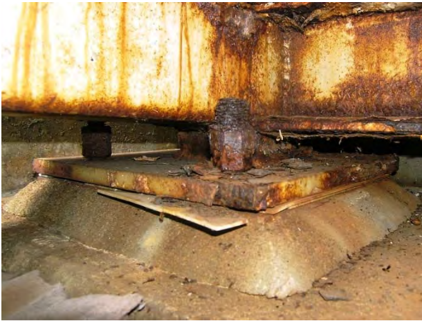
Left Bearing – North Abutment- Expansion
