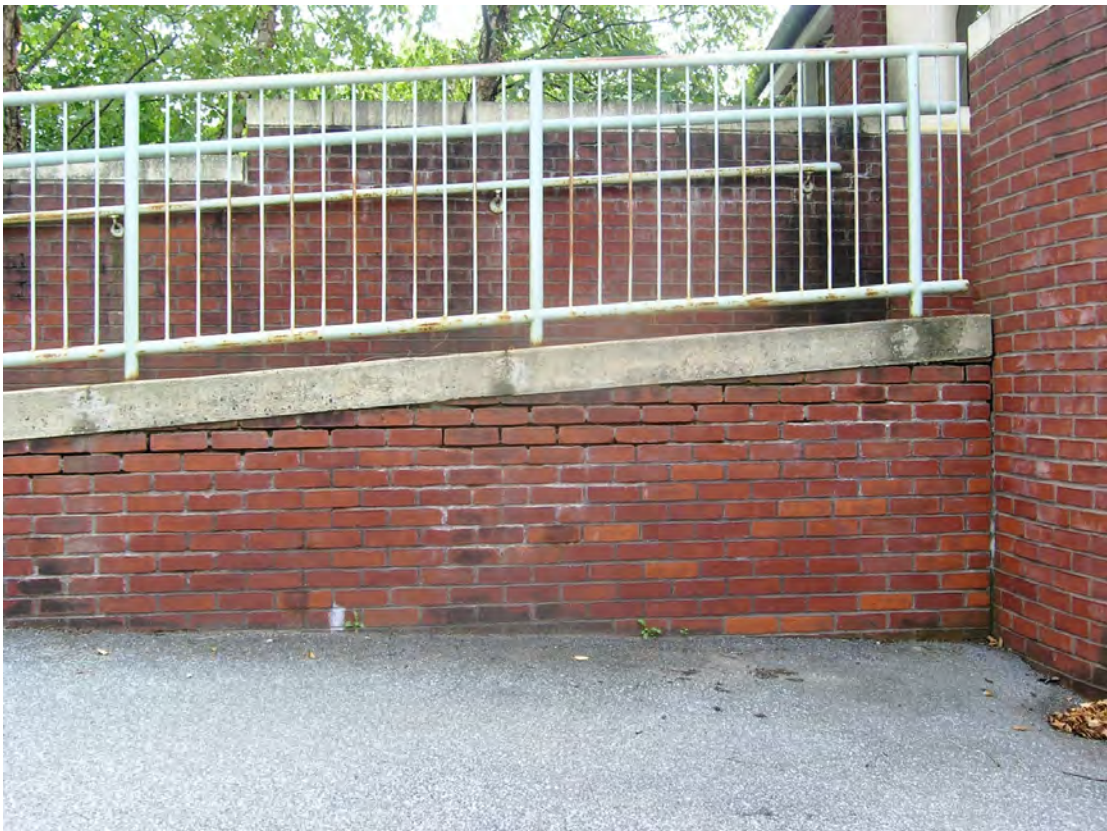
19) Loss of pointing below ramp at Wing Wall D, north approach
