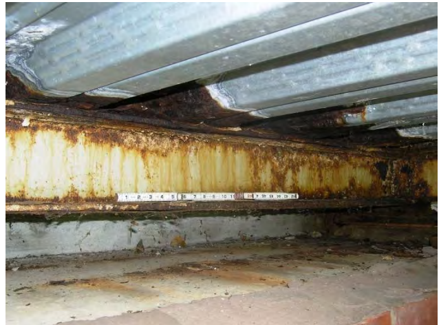
Typical Condition – End Floorbeam
