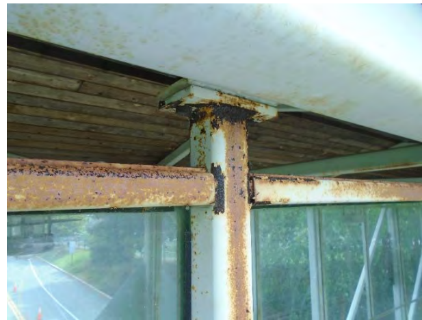
Typical Condition – Top of Plexiglass Support
