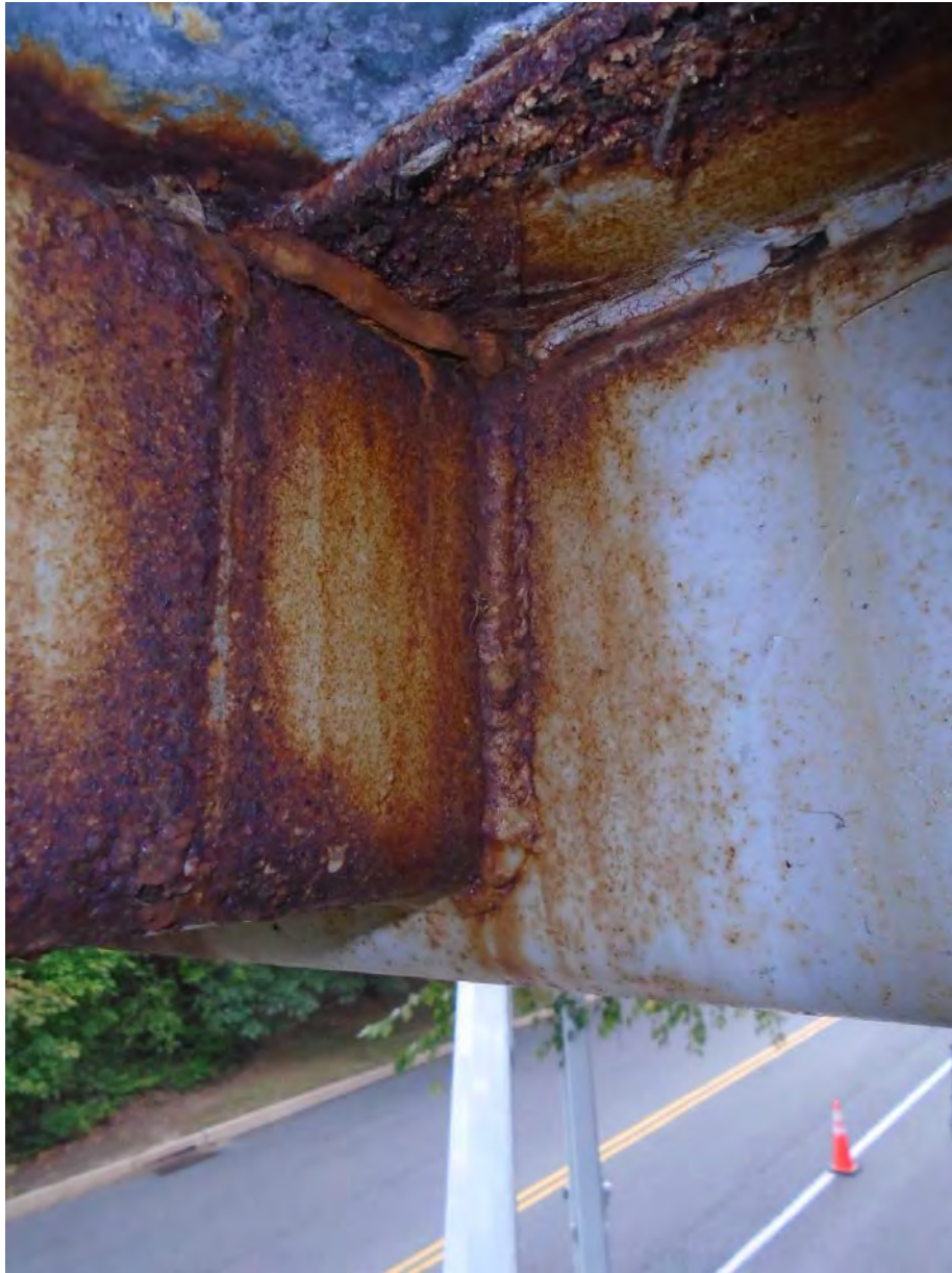
5) Typical connection of floorbeam to bottom chord
