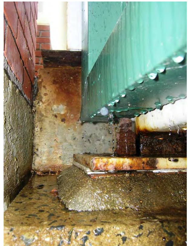
Water Leaking from Downspout Seams onto the Bridge Seat – Typical
