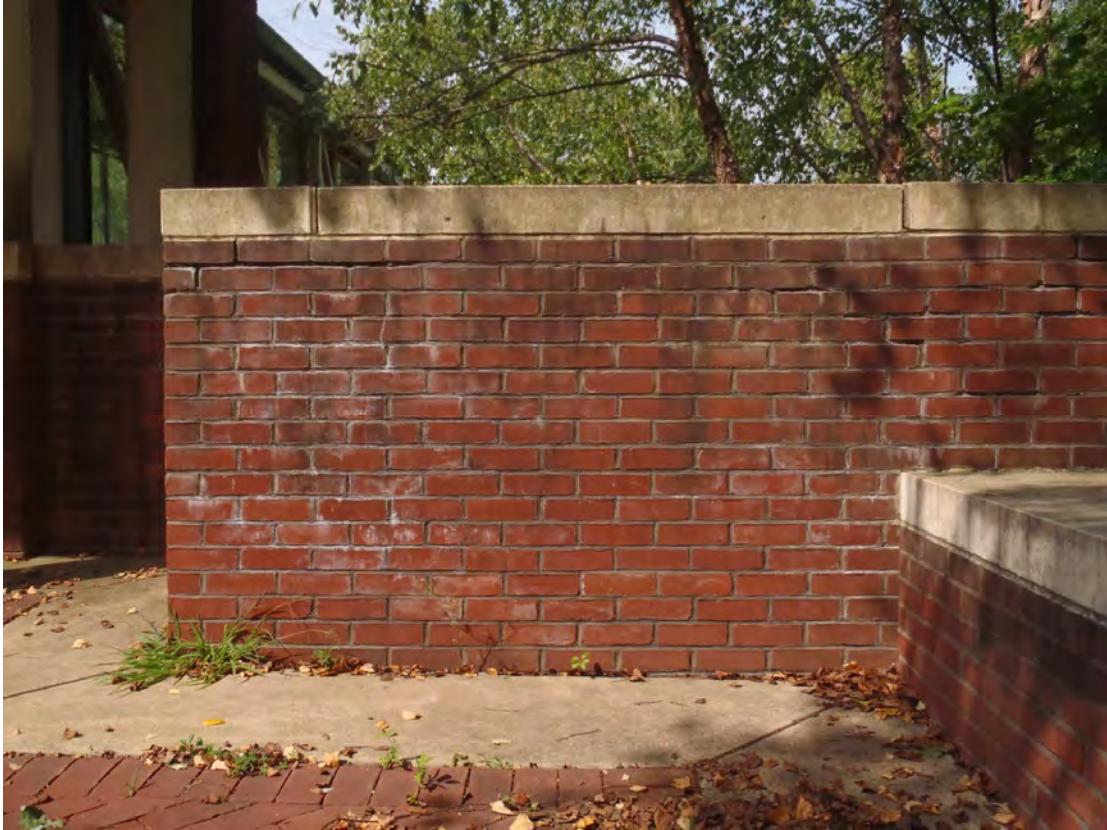
20) Wing Wall A, rear face parapet—Typical condition, areas of missing pointing and efflorescence
