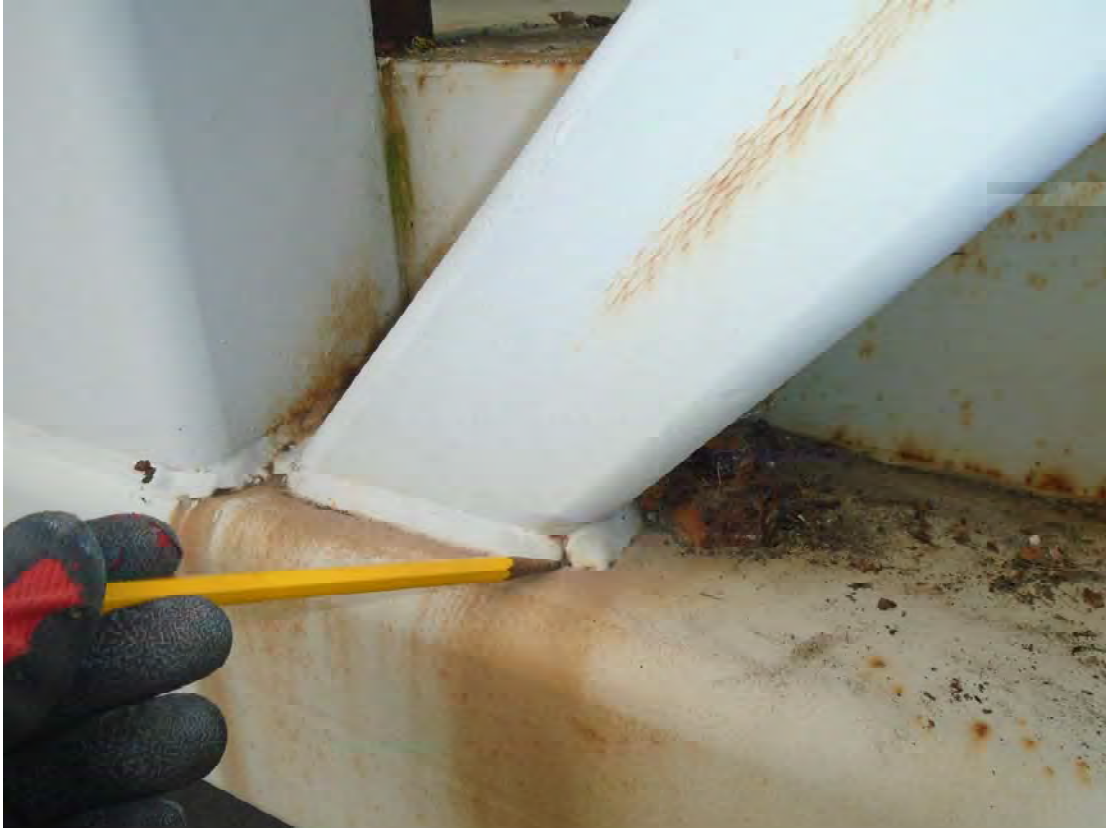
3) Discontinuous weld at L5-U6 at bottom chord
