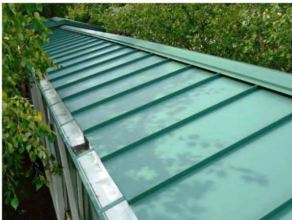
Typical Condition – Standing Seam Metal Top
