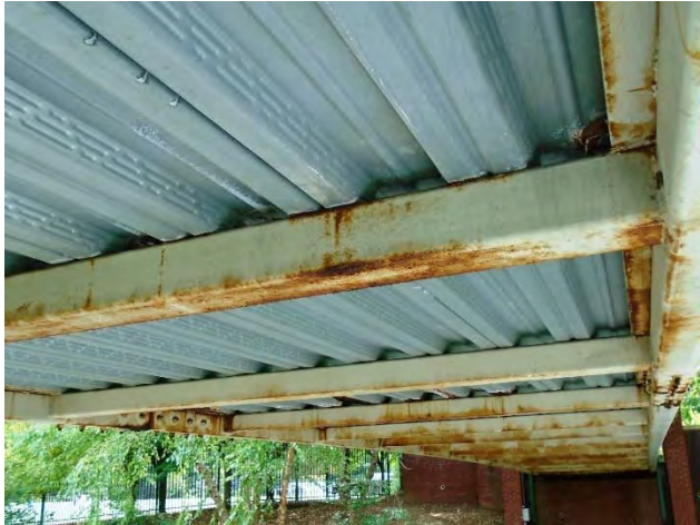
Typical Condition - Floorbeam
