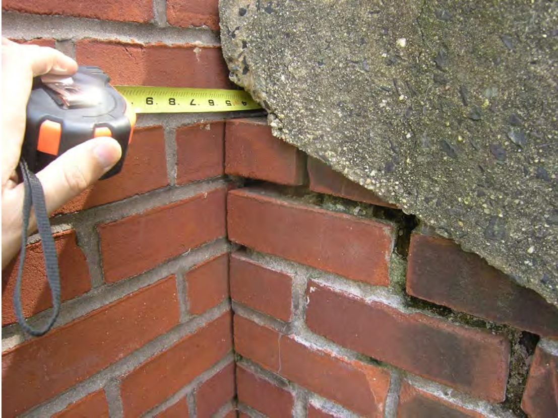
18) Loss of pointing below stairs at Wing Wall C, north approach
