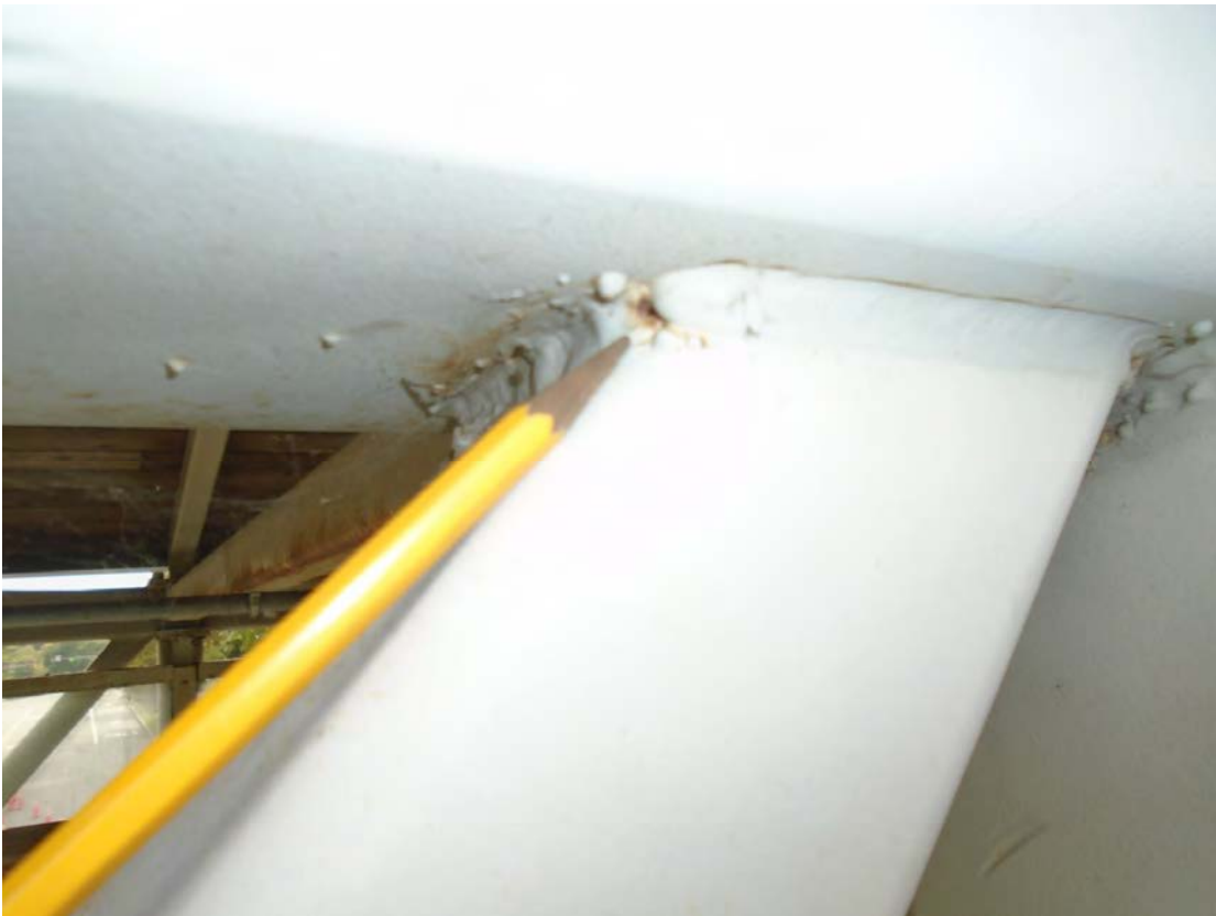
2) Typical welds to top chord
