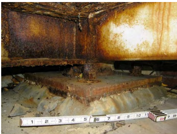
Left Bearing – South Abutment: Fixed
