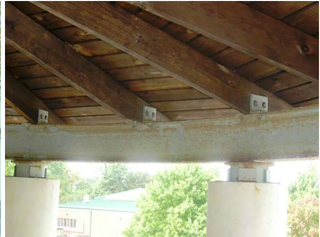
Typical Condition of Portico Curved Steel Support Beam
