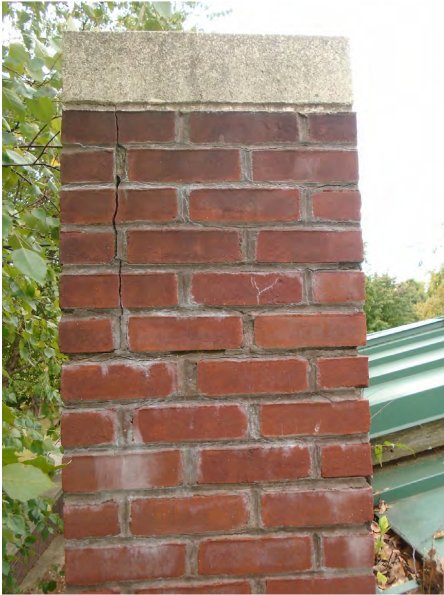
24) Cracked brick & pointing at Near (South) right pillar (looking South)
