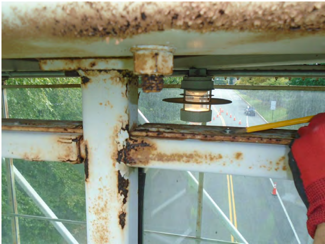
4) Loose connector at Panel Point 5.5
