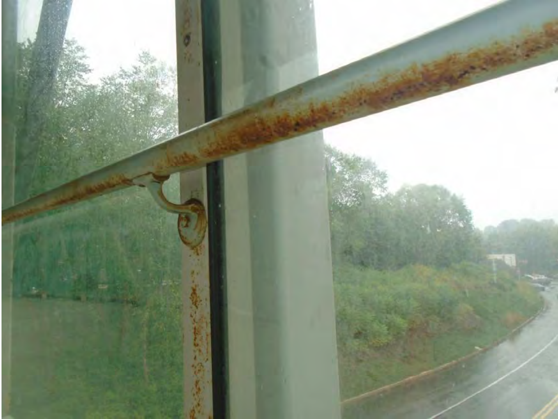
31) Typical railing condition and connection to glass framing support
