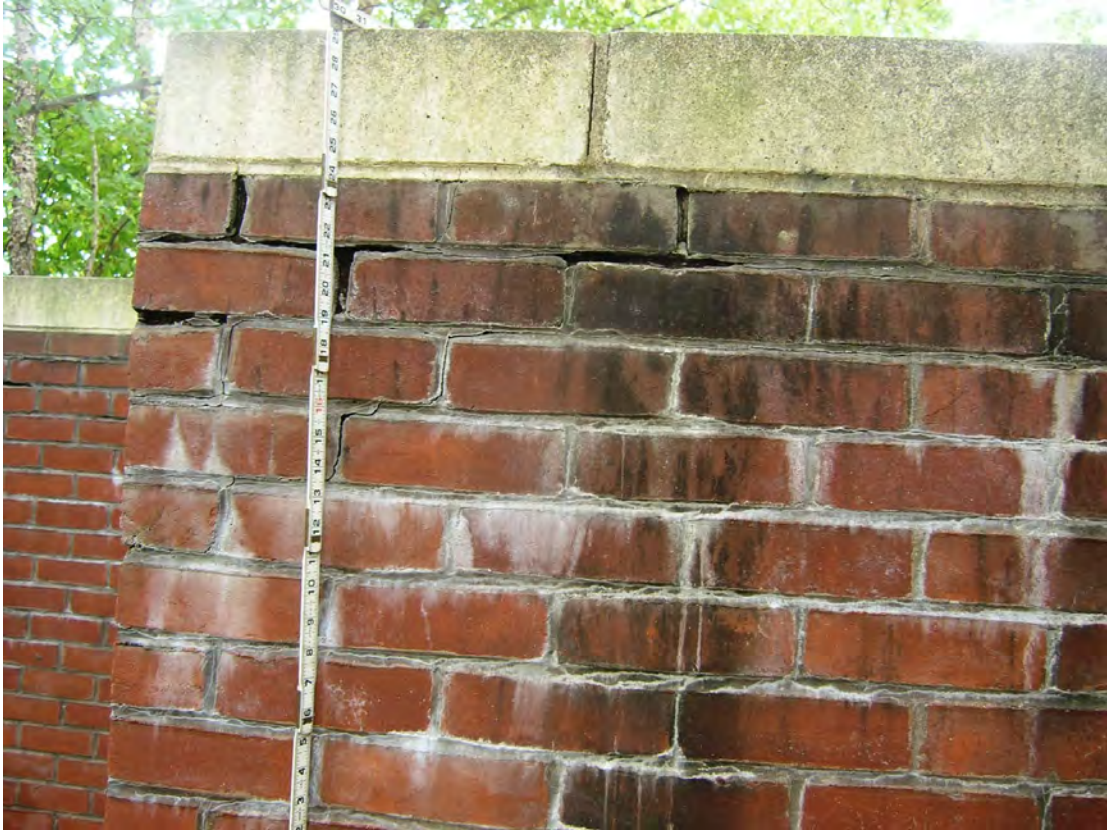
16) Detail of location with missing and cracked pointing—Wing Wall A
