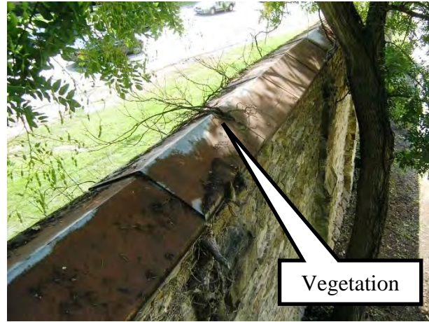
General View of Intact Roof Cap Showing Minor Surface Rust and Vegetation Growing from the Joints in the Metal Sheathing
