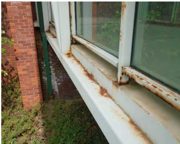
Typical Rust/Blisters on Top of Bottom Chord
