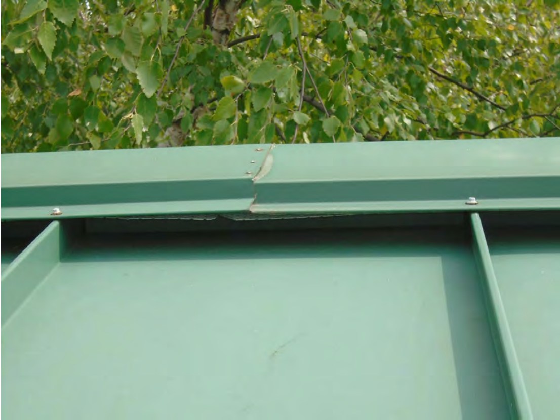
27) Separation in roof ridge line cap near Panel Point 8
