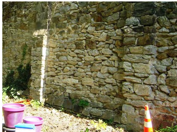
Typical Missing Mortar & Loose Base Stones
