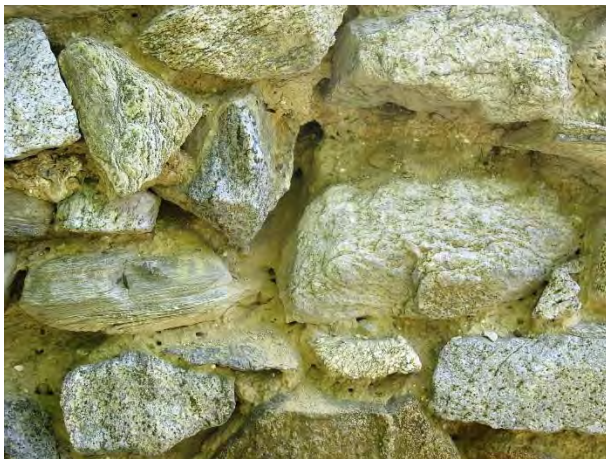
Detail of Deteriorated and Sandy Mortar
