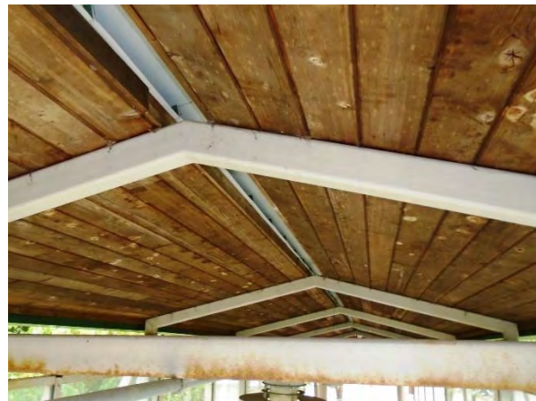
Typical Condition – Timber Roof Planking
