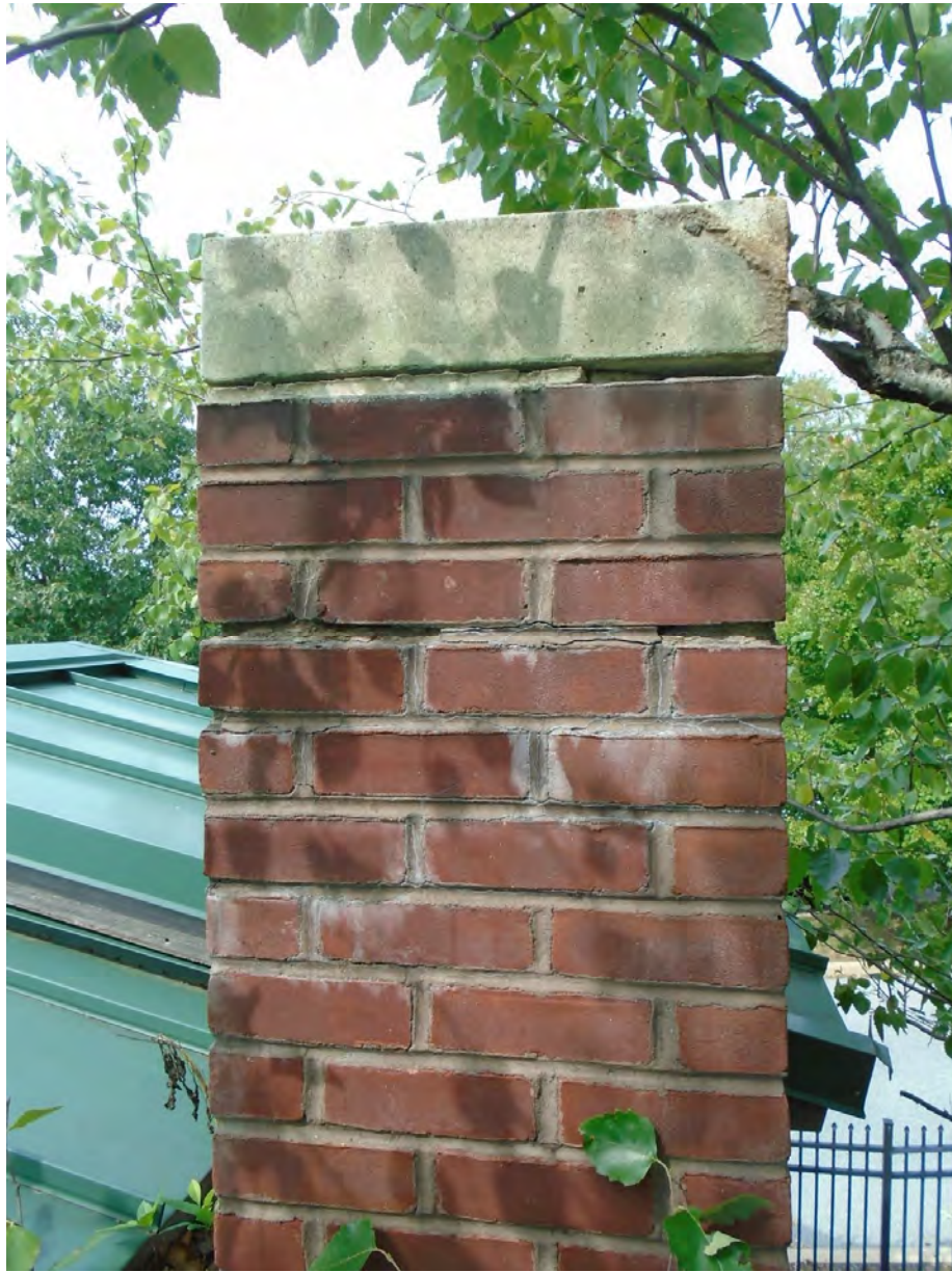
25) Loose/missing pointing at far (north) right pillar (looking north)
