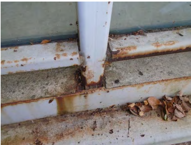
Typical Condition – Bottom of Plexiglass Support
