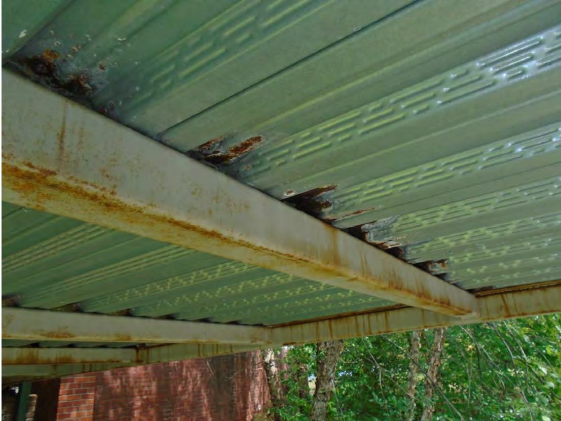
6) Rusted, delaminated deck forms over Floorbeam 8 (typical FB9)
