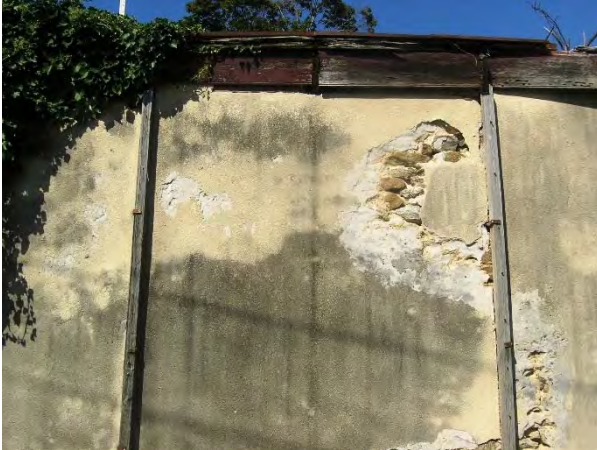
Typical Condition of Pargeted Surface and Vertical Timbers on East Face
