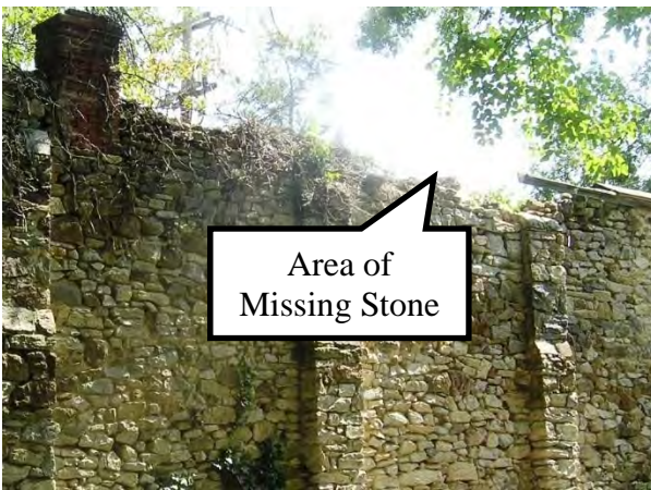
Area of Missing Stone Along Top Face of Pilaster Wall
