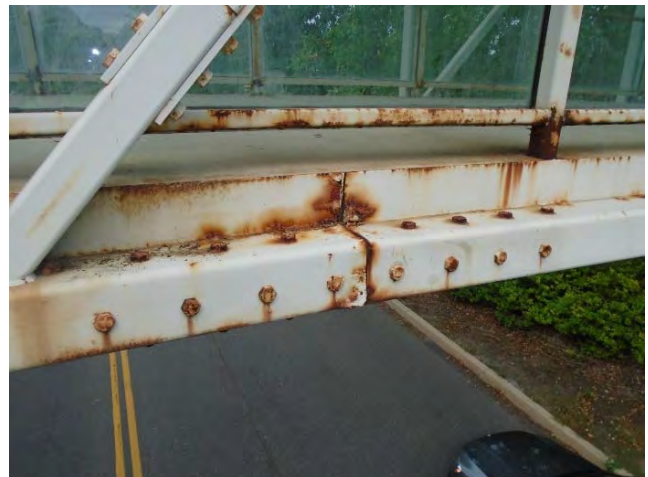
Typical Rust & Peeling Paint at Midspan Splice
