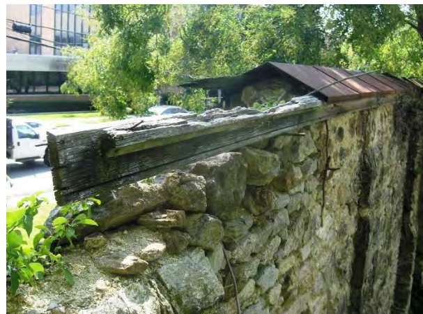
Deteriorated, Broken and Missing Roof Cap
