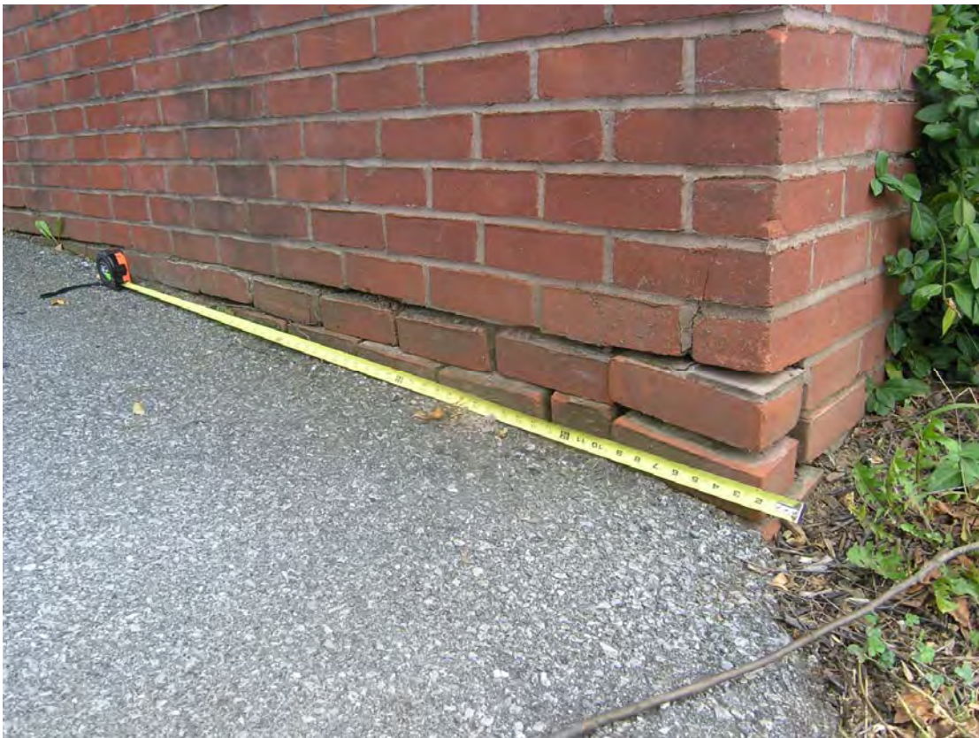
17) Loose bricks at end of Wing Wall C, near face
