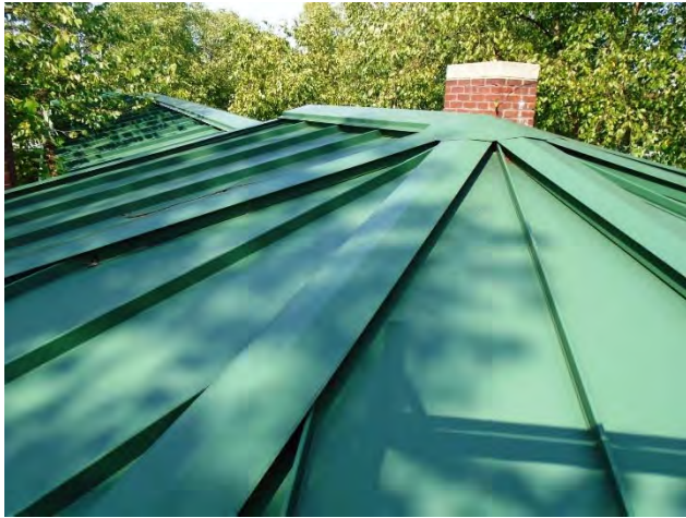
General View and Typical Condition of Portico Standing Seam Metal Roof
