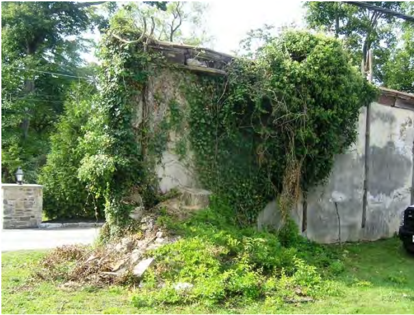
Heavy Vegetation Growth and Failed South End Wall, South End of Pilaster Wall
