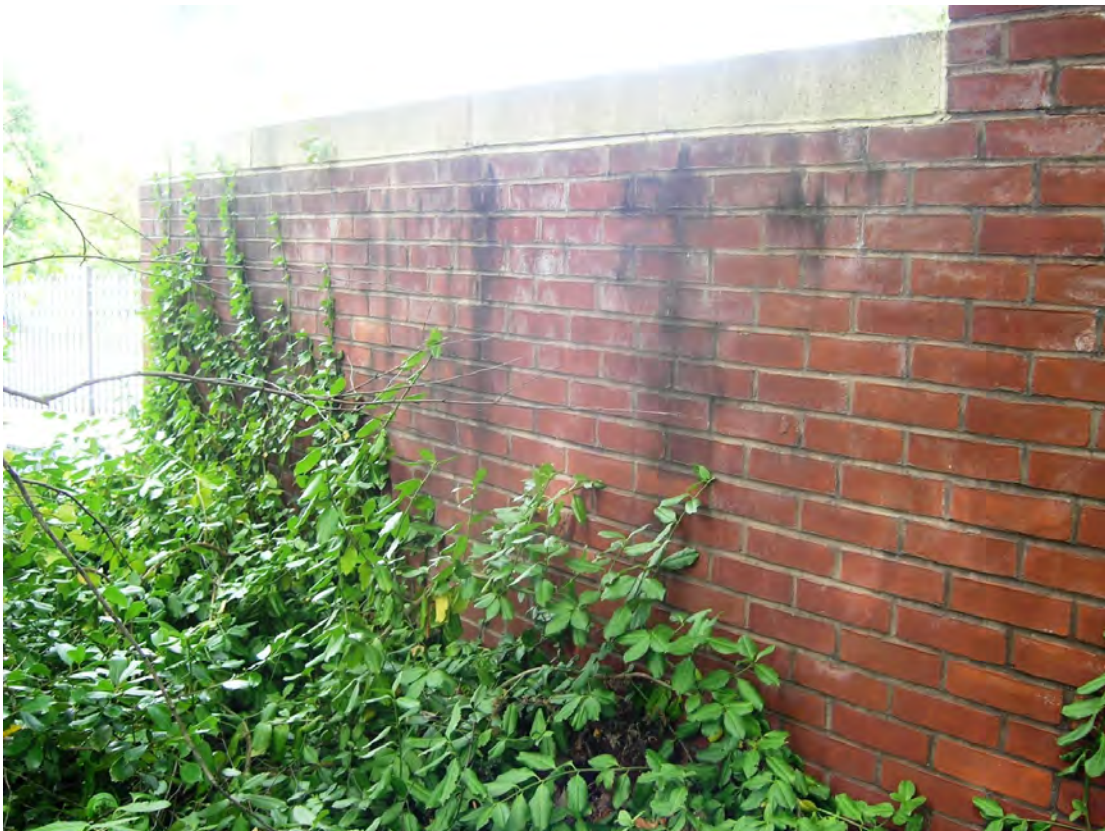
14) Wing Wall C—General view of west end of wing wall with vegetation growth
