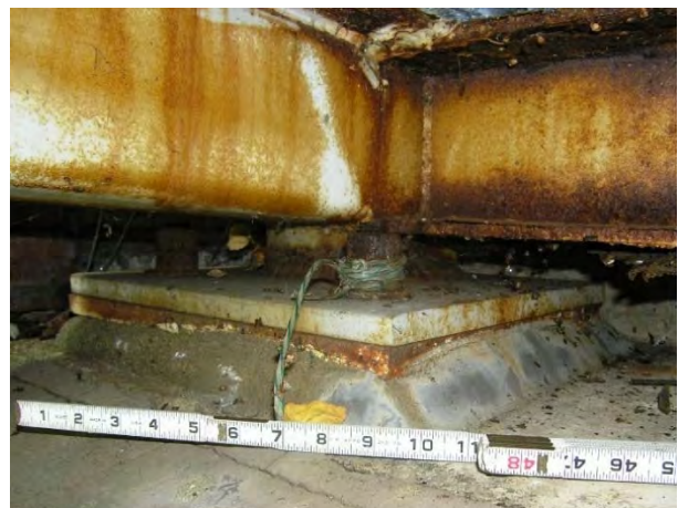
Right Bearing – South Abutment: Fixed
