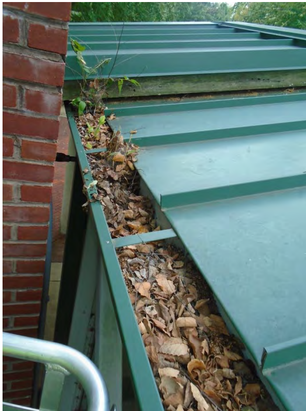
Debris Clogging Gutters
