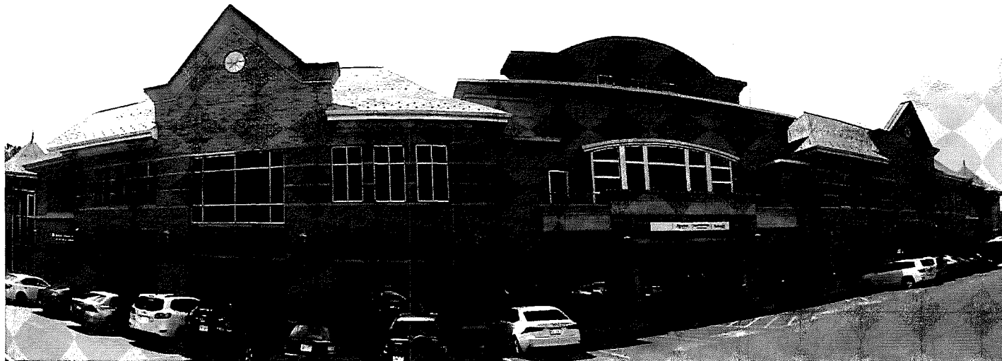
9 Back of Building (North Facade, Photo Provided on 12/10/15) scale: n.i.s.
