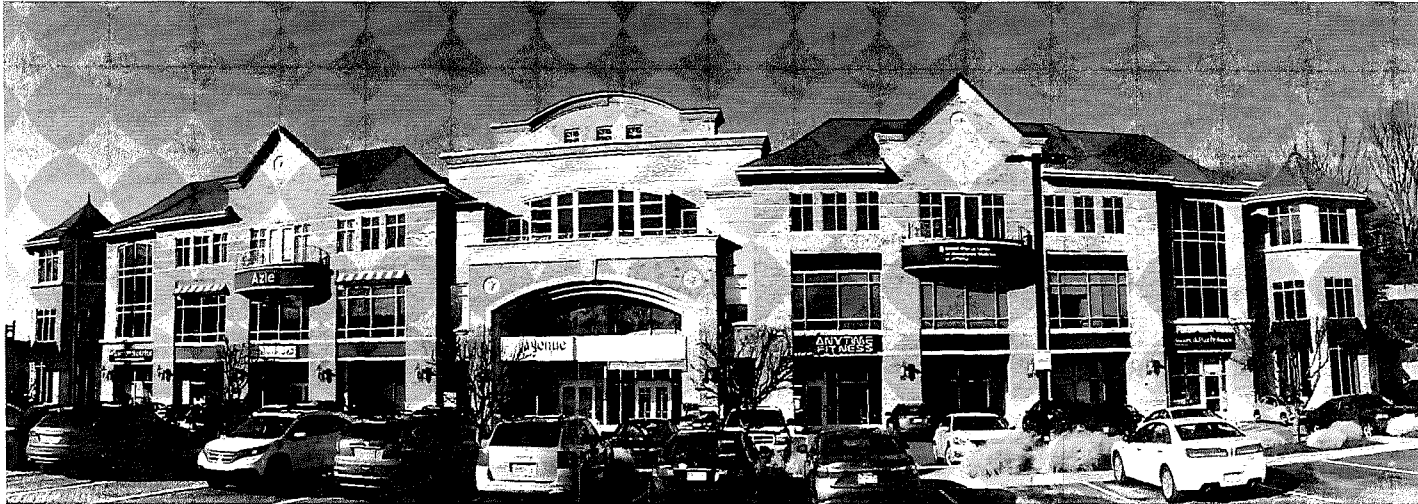
8 Front of Building (South Facade, Photo Provided on 03/07/16) scale: n.i.s.
