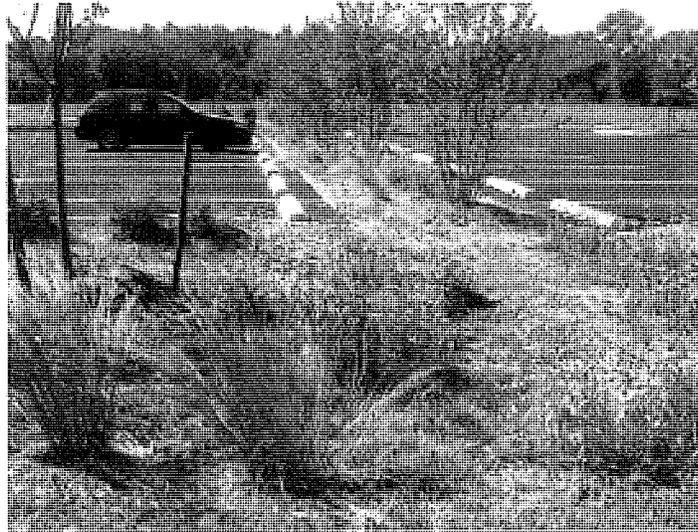
Designed and constructed in accordance with Pennsylvania Stormwater Best Management Practices Manual guidelines, this project stores an estimated 9170 cubic feet of stormwater and treats an estimated 85% of total suspended solids, 85% of phosphorous, and 30% of nitrates from stormwater runoff discharging to Towamencin Creek.
