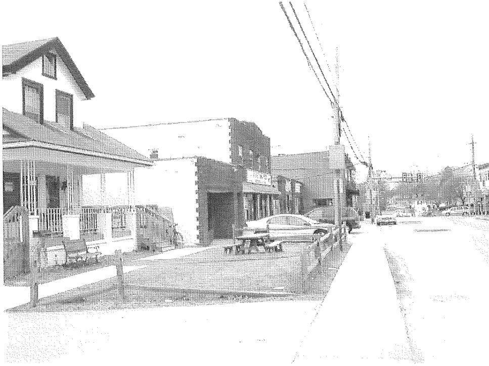
Existing condition of facades
