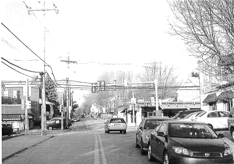
Existing condition of Garrett Avenue
