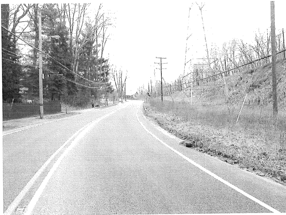
Existing condition of the eastern gateway
