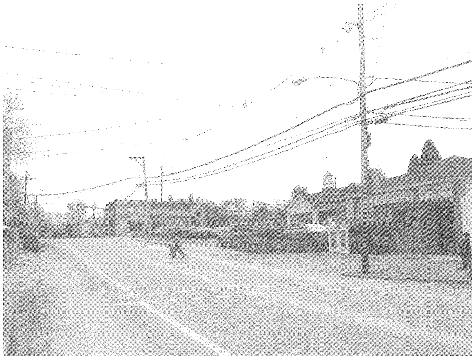
Existing conditions on Conestoga Road
