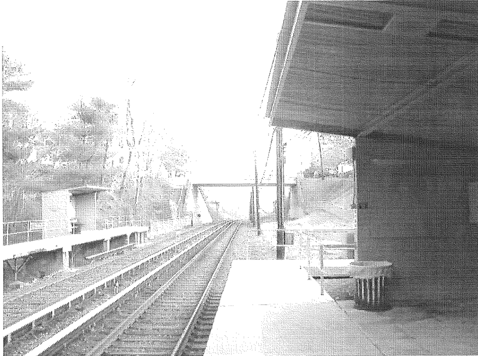
Existing conditions at the Route 100 station
