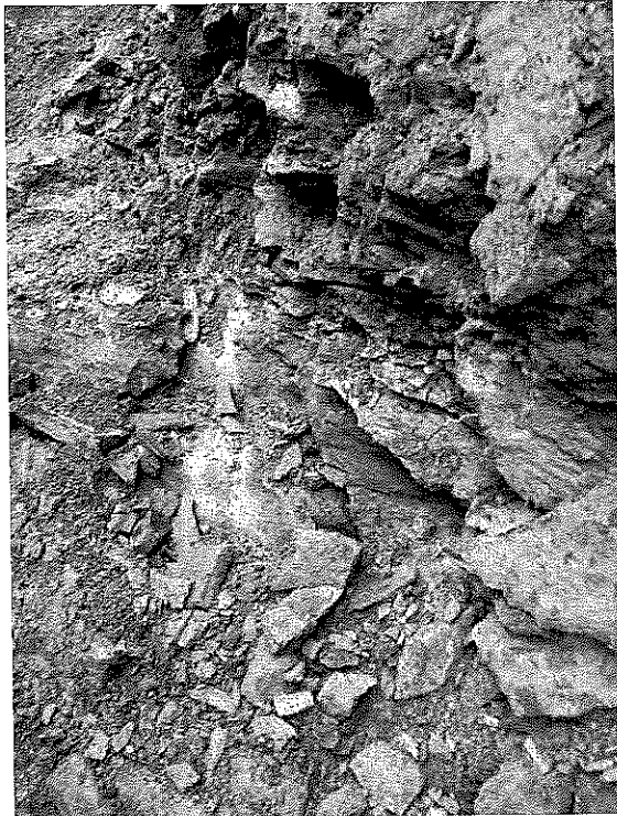
Test Pit #SWM-04 at 39 inches
