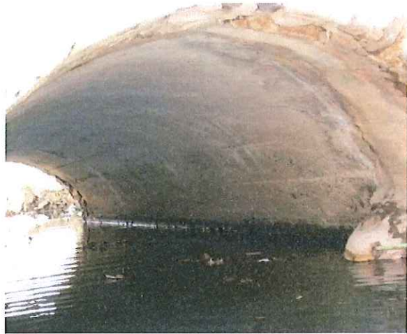
View of Concrete Arch North Barrel
