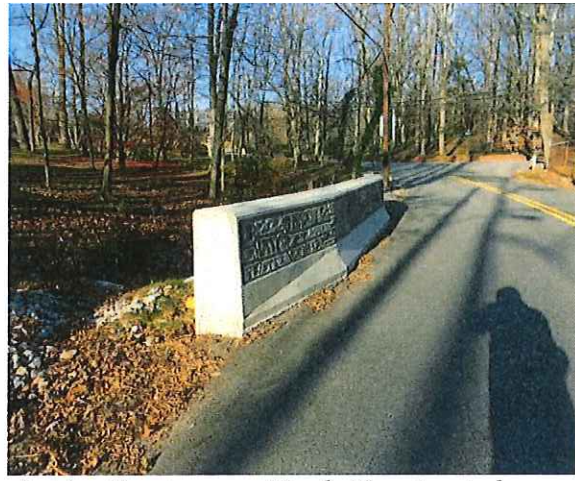
Bridge Barrier on a Newly Constructed Bridge along Chamounix Road over Branch of Gulph Creek
