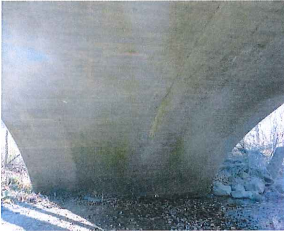
Concrete Arch Barrel – Looking at West Abutment
