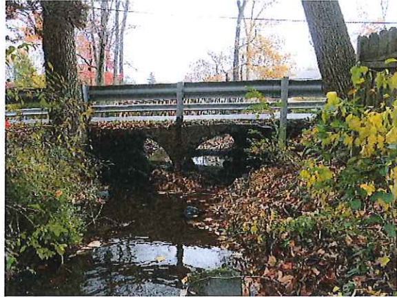
North Grouted Masonry Headwall
