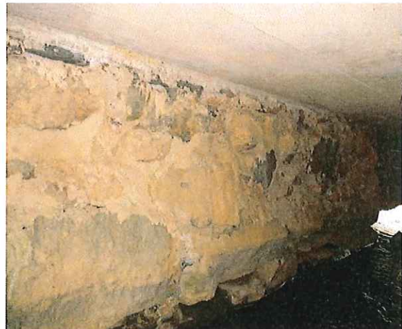
View of Original South Stone Masonry Abutment
