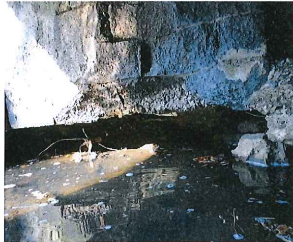
North Abutment of Inlet Structure – Looking Southwest
