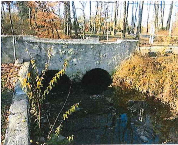
Downstream Retaining Wall – Looking Upstream
