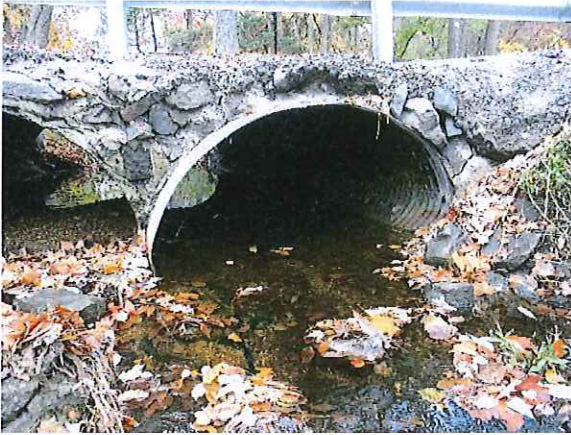
South Grouted Masonry Headwall
