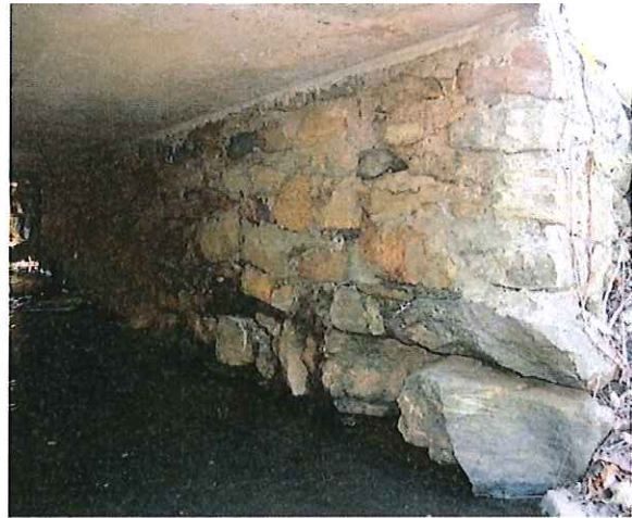
View of Original North Stone Masonry Abutment
