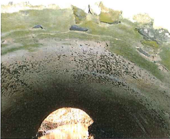
View of Concrete Arch South Barrel
