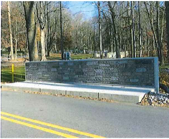
Sidewalk on a Newly Constructed Bridge along Chamounix Road over Branch of Gulph Creek
