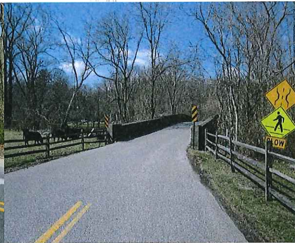
East Approach, Note Sign of Pedestrian Crossing
