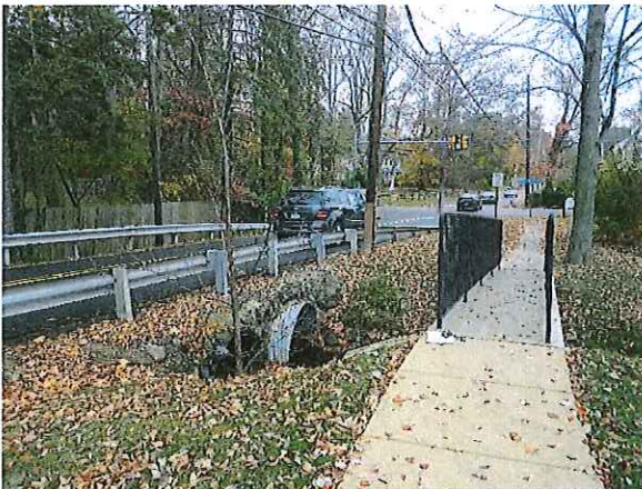
General View of Culvert and Pedestrian Bridge
