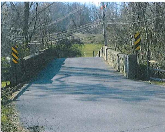
General View of Arch Bridge – Looking East
