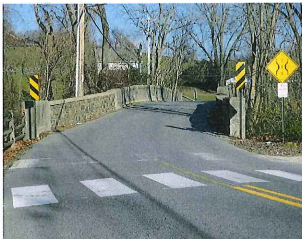
West Approach, Note Pedestrian Cross Walk was Previously Relocated Once
