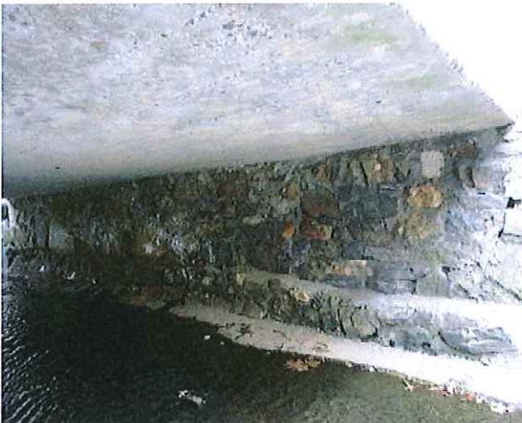
Typical Masonry Abutment
