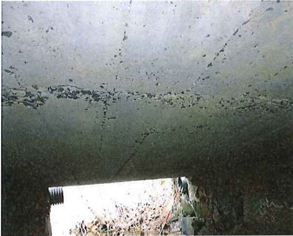
Under Deck View (H.C. in middle width)
