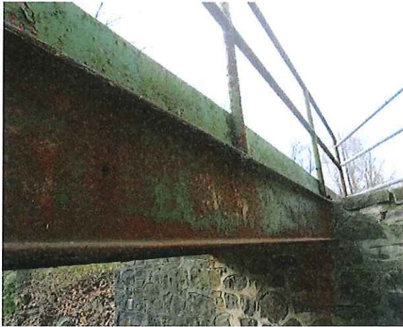
South Pedestrian Bridge Elevation View
