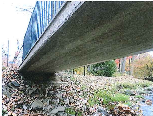
Underdeck View of Pedestrian Bridge
