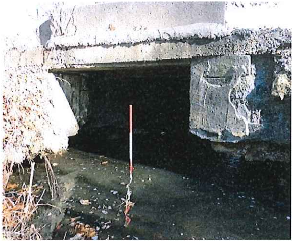
West Fascia - Inlet Structure
