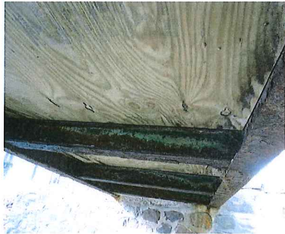
South Pedestrian Bridge Underdeck View
