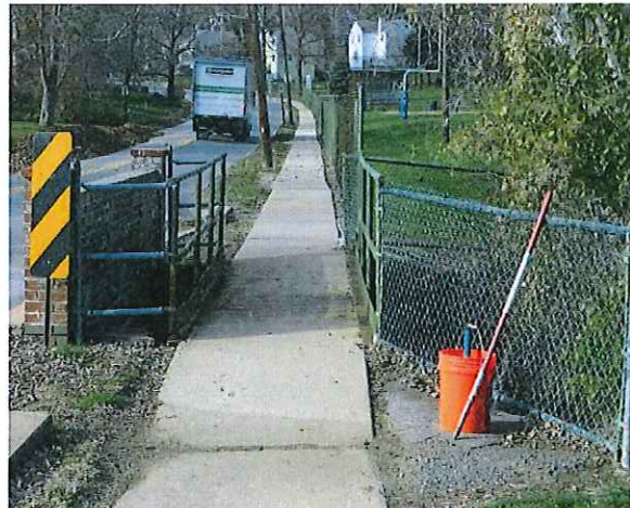
North Pedestrian Bridge (South Pedestrian similar)
