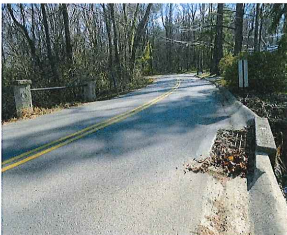
General View of Culvert – Looking South. Note Inlet Structure in West Shoulder
