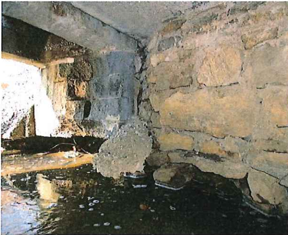
North Abutment of Inlet Structure – Looking Northwest
