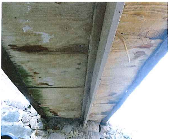
North Pedestrian Bridge Underdeck View
