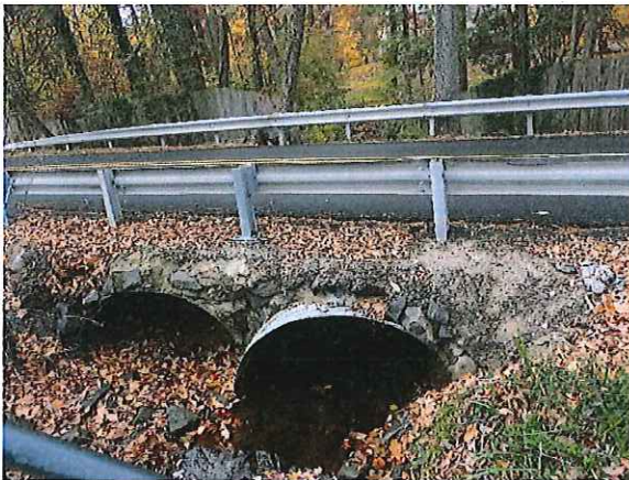
Guiderail Posts at South Fascia
