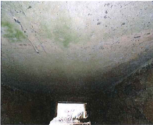
View of Original Concrete Slab Superstructure (underside)
