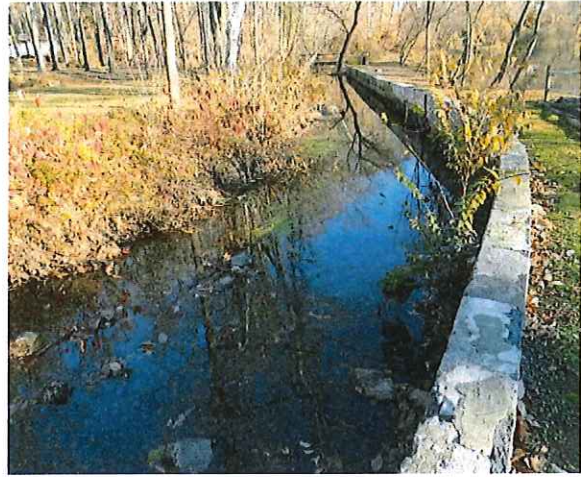
Downstream Retaining Wall – Looking Downstream
