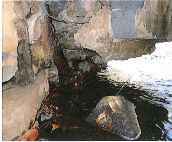
South Abutment of Inlet Structure – Looking Southwest
