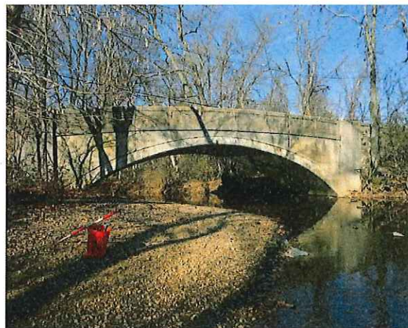
Downstream (South) Elevation
