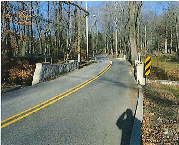
General View of Culvert – Looking North
