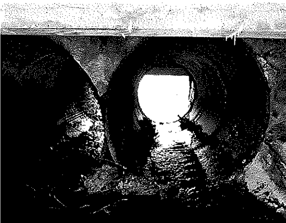
Culvert Inlet ~ 6" deep
