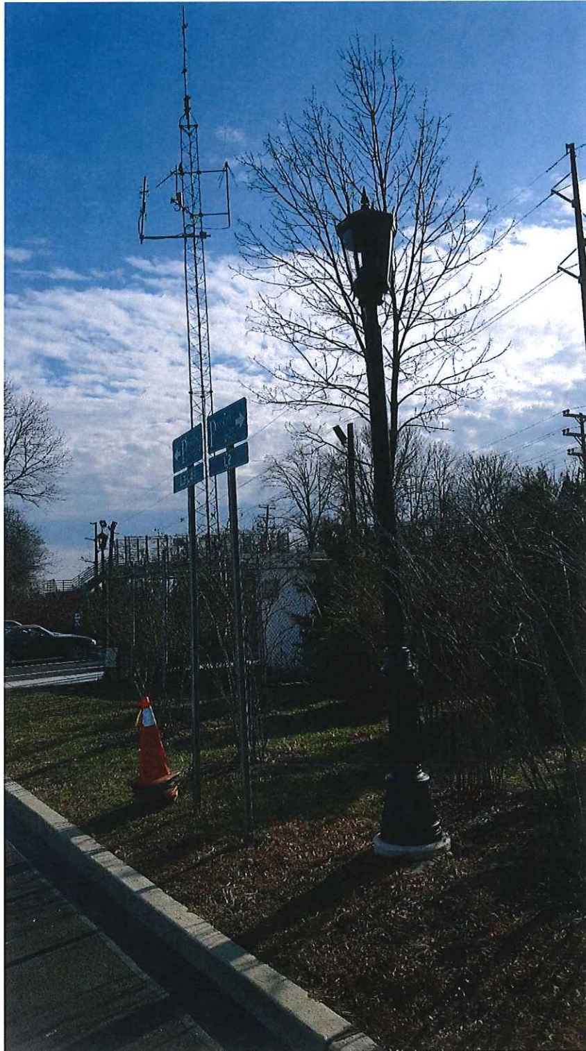
Site photo, typical WLAPF luminaire with full cut-off shield
