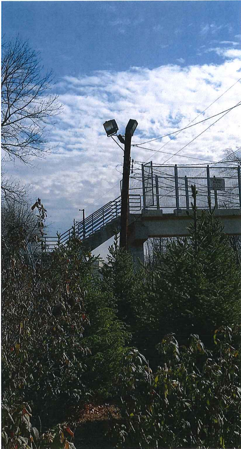
Site photo, typical SEPTA NHSL station pole-mounted luminaire
