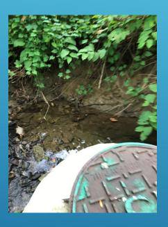
When originally constructed, this manhole was ten feet into the stream bank. Over the years, erosive forces have eroded the stream bank, and the manhole, as well as the concrete encasement are exposed in the stream. The pipe repair will pale in comparison to the permitting and stream bank restoration costs. This project is requested in the 2018 sanitary sewer capital budget, titled Rawles Run.
