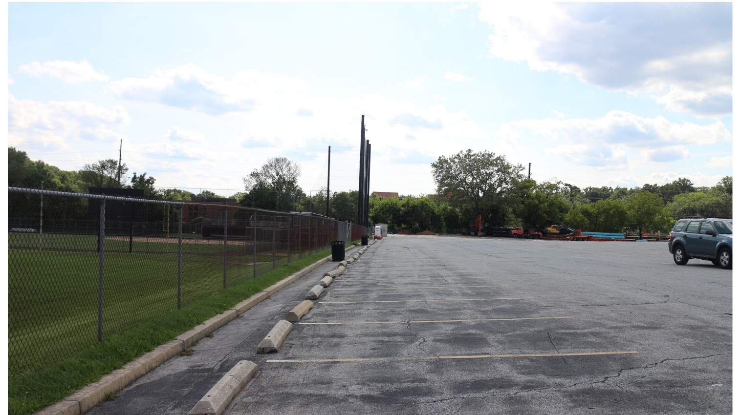
VIEW FROM MAIN LOT PARKING LOOKING SOUTH
