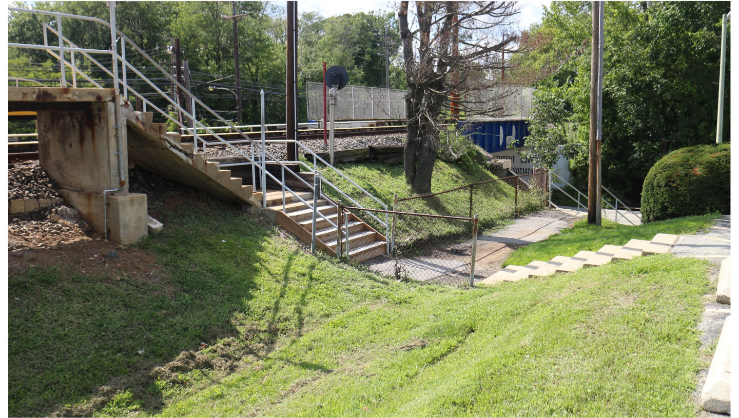
STADIUM STATION STAIRS AT NORTH SIDE OF RR
