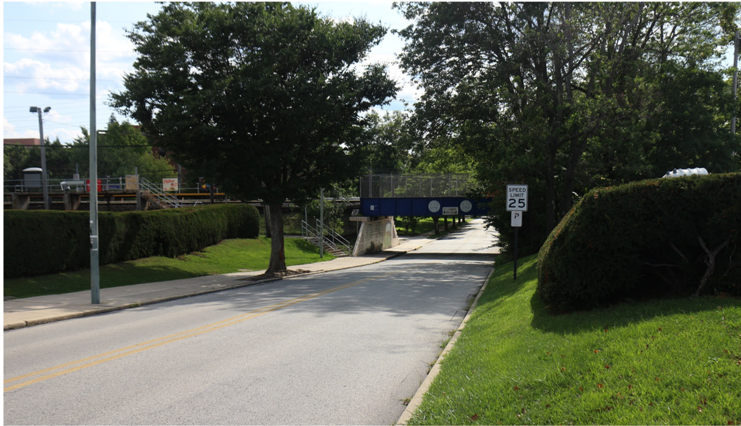
VIEW OF RR BRIDGE FROM ITHAN AVENUE LOOKING SOUTH
