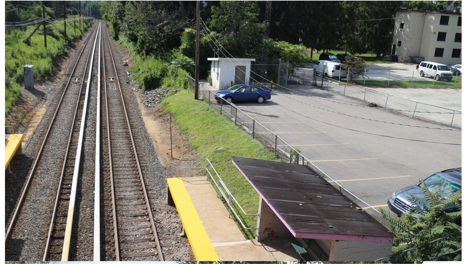
VIEW OF MAIN LOT PARKING LOOKING SOUTH WEST
