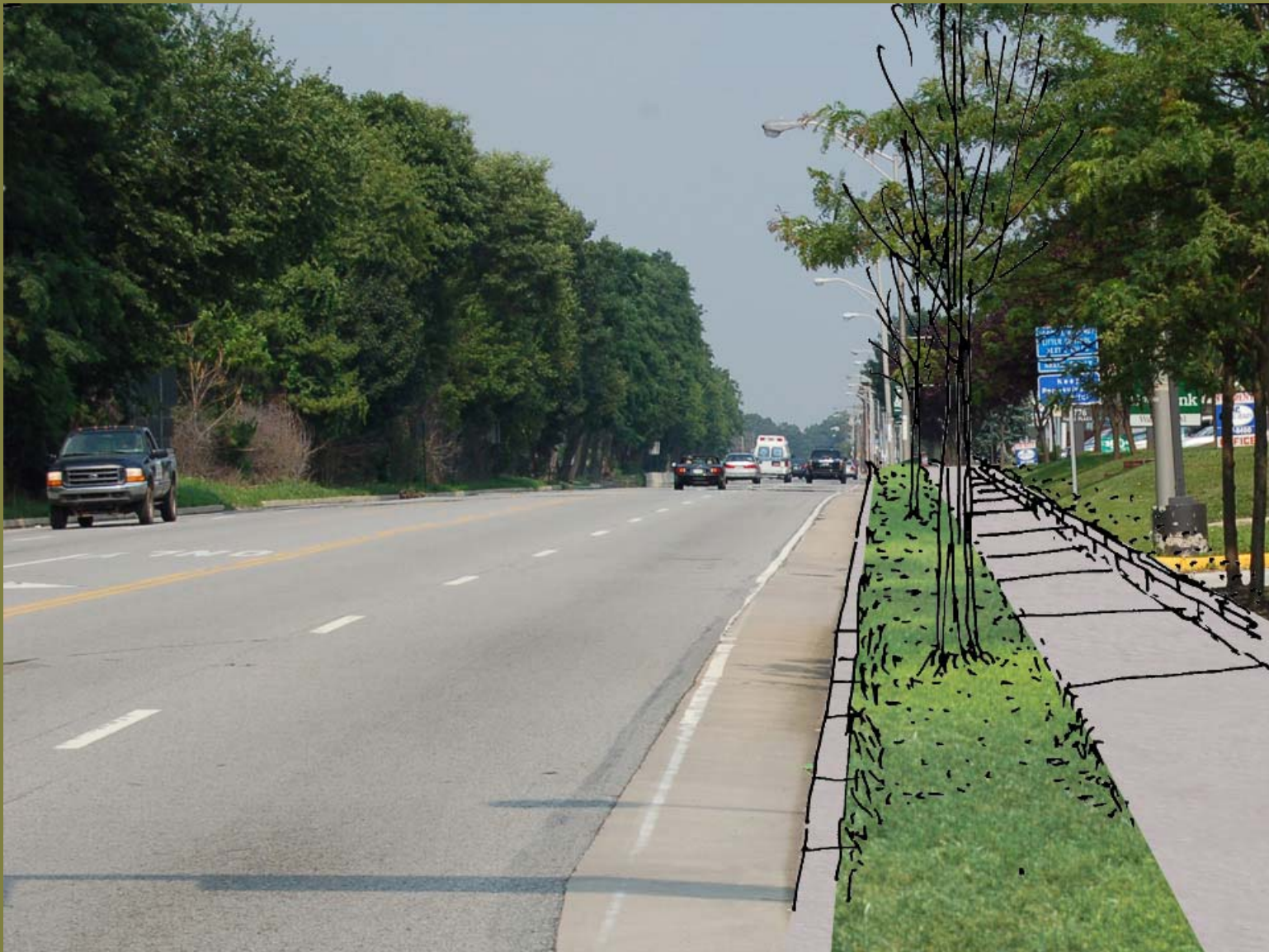
Sidewalk, south side of Lancaster Avenue near Leopard Road
