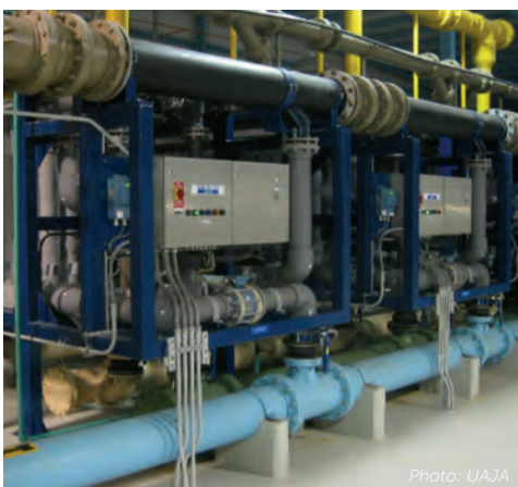
UAJA Beneficial Reuse Project purifies wastewater through micro-filtration and reverse osmosis used to augment Slab Cabin Run and recharge the drinking water aquifer.
