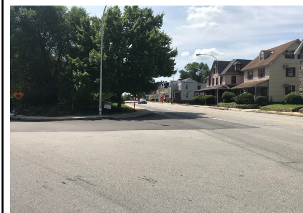
Photo 9: Westbound Old Lancaster Rd, looking left.
