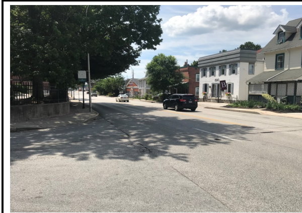
Photo 11: Westbound Mondella Ave, looking left.
