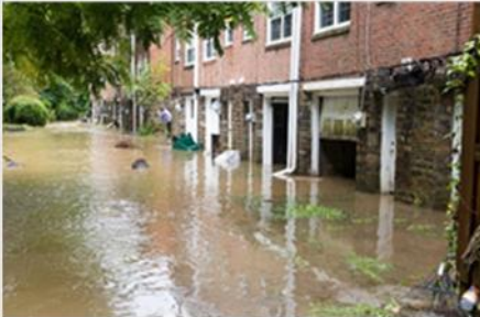
Flash flooding in Radnor Township August 2018
